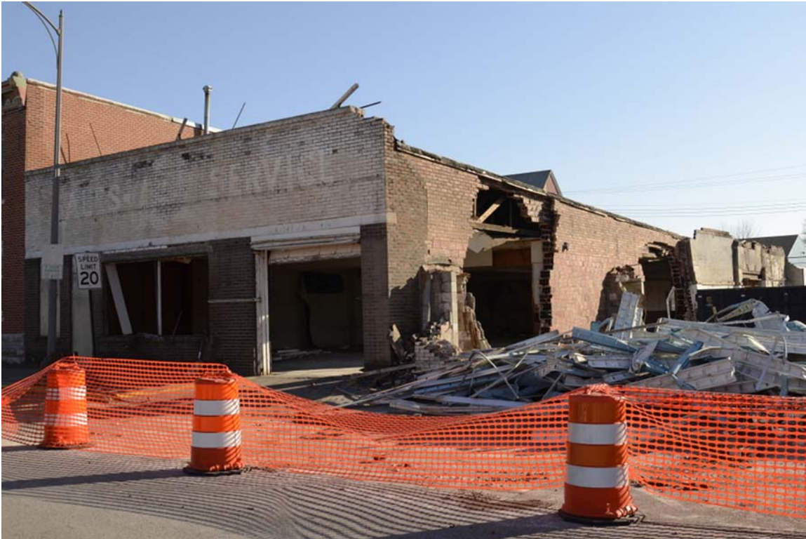
Photograph 92-00612-002 - North and west elevations of 215-217 W. Washington, looking southeast (December 2, 2010)
