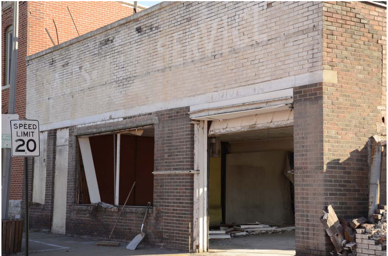
Photograph 92-00612-003 - North elevation of 215-217 W. Washington, looking southeast (December 2, 2010)
