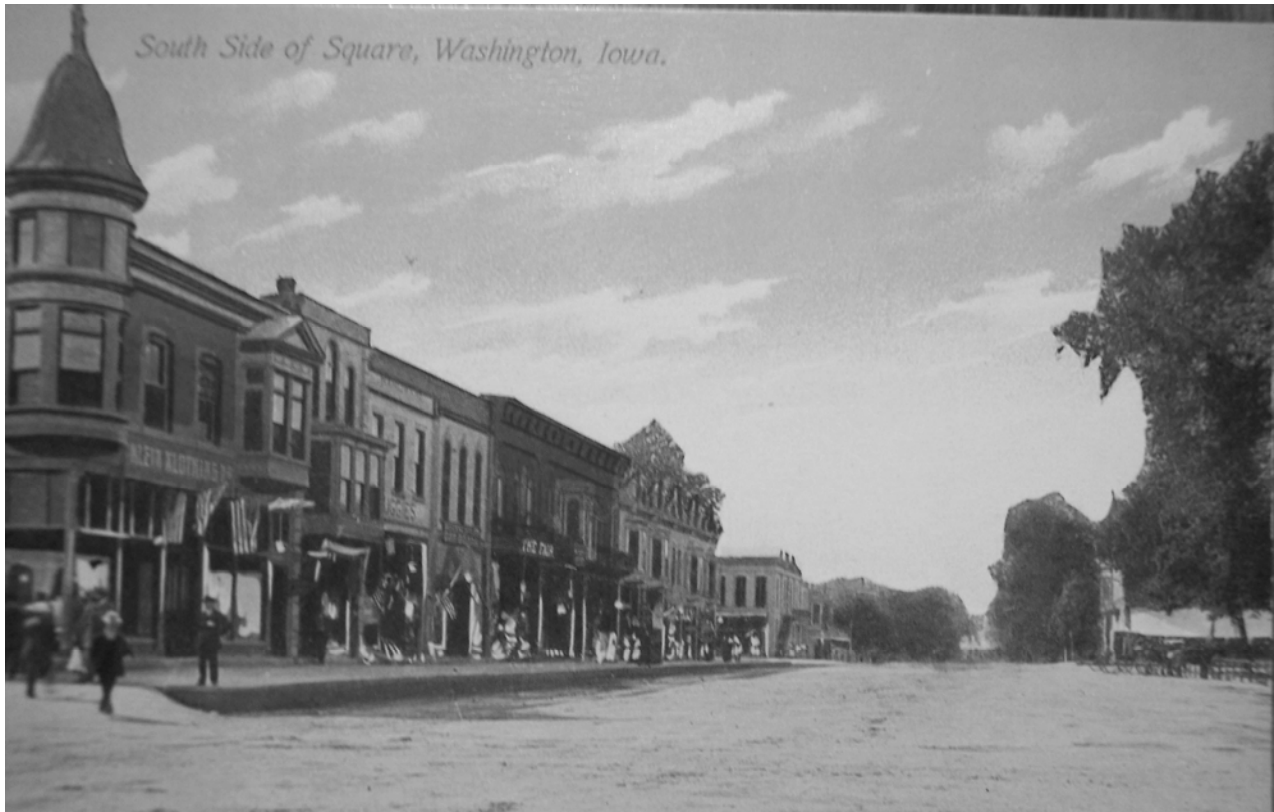
Figure 37. South side of square (100 block of W. Washington) in early 1900s, looking west (Patterson collection).
