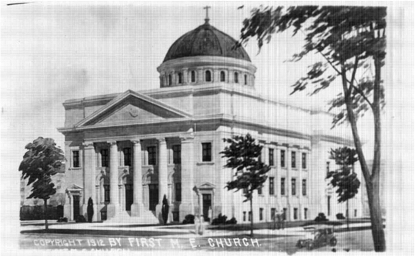
Figure 45. Methodist Episcopal Church at 206 W. 2 nd Street built in 1912-14 (Map #12) (Patterson collection).
