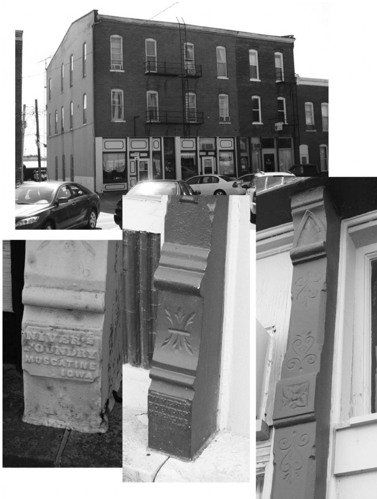
Figure 19. Kerchner Block built in 1892, detail of storefront columns from Niver's Foundry (Map #5) (McCarley 2011).
