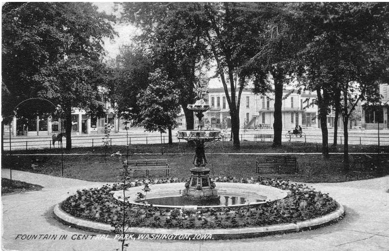
Figure 30. Central Park in 1910, looking southwest at fountain (Map #100) (Patterson collection).
