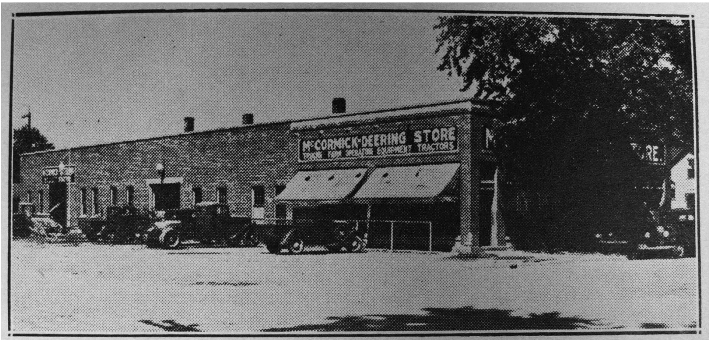
Figure 63. Piper Garage (later Washington International Company, and then McCormick-Deering Store) built around 1925 at 102 E. 3 rd Street (Map #38) ( Evening Journal , July 1936, 24).
