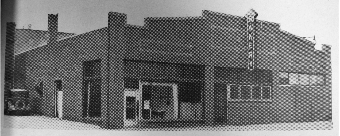
Figure 62. Garage built in early 1920s at 107-109 W. 2 nd Street (Map #46), converted around 1931 for H & A Baking Company ( Evening Journal , July 1936, 95).
