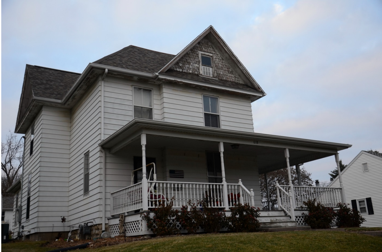
Figure 29. Adam Wombacher House at 618 W. Main Street (December 2014).
