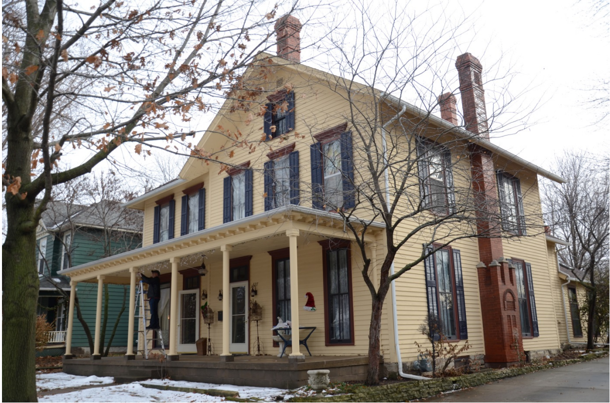
Figure 13. Burrell House at 527 W. Washington Blvd (December 2014).
