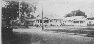
Stucco Cottages on South Iowa Ave., built by Charles Schnoeller
