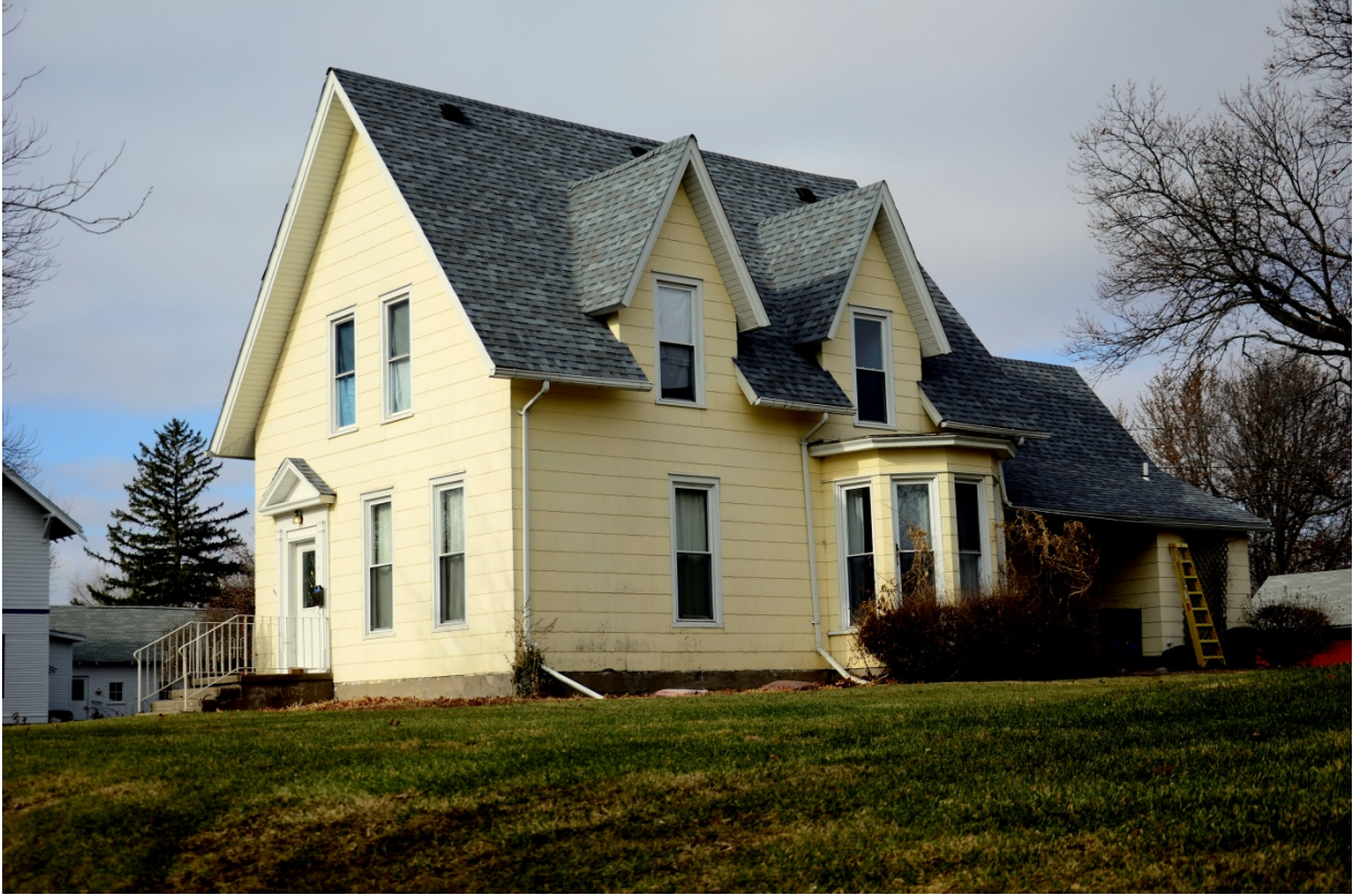
Figure 8. Sanford House at 714 W. Main (December 2014).
