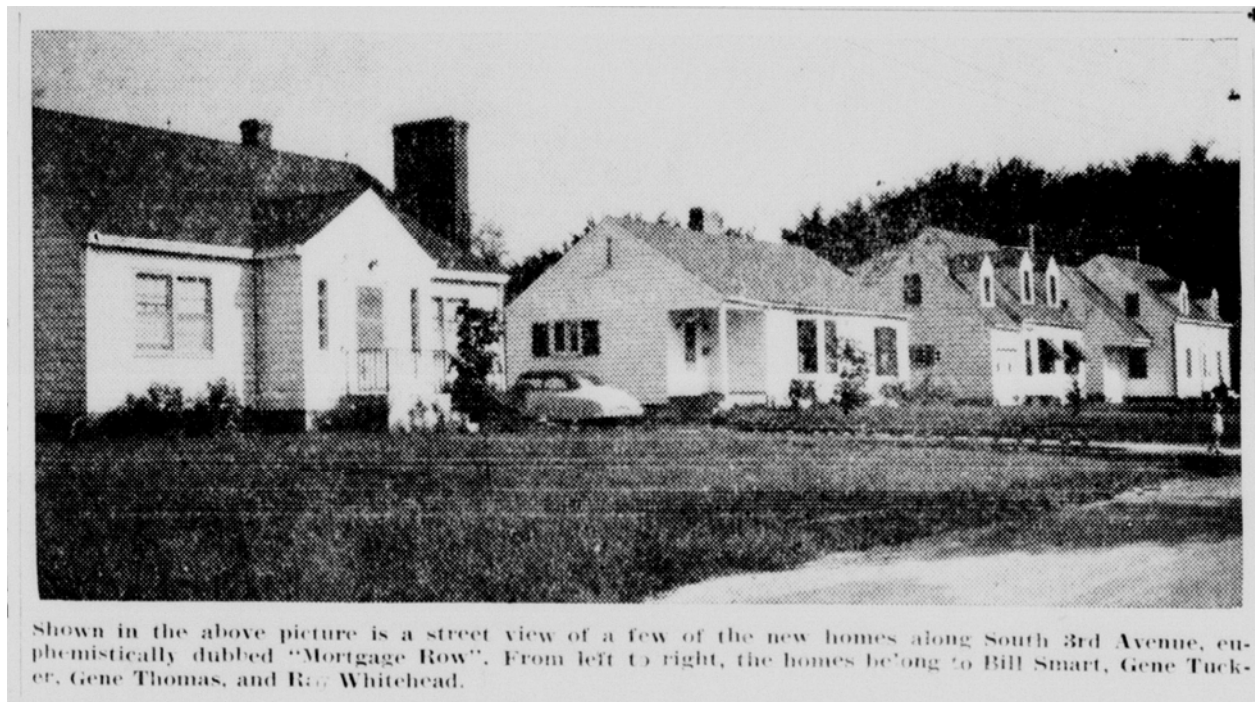
Figure 56. Houses along S. 3 rd Avenue in 1949 ( Evening Journal , August 19, 1949, 7).
