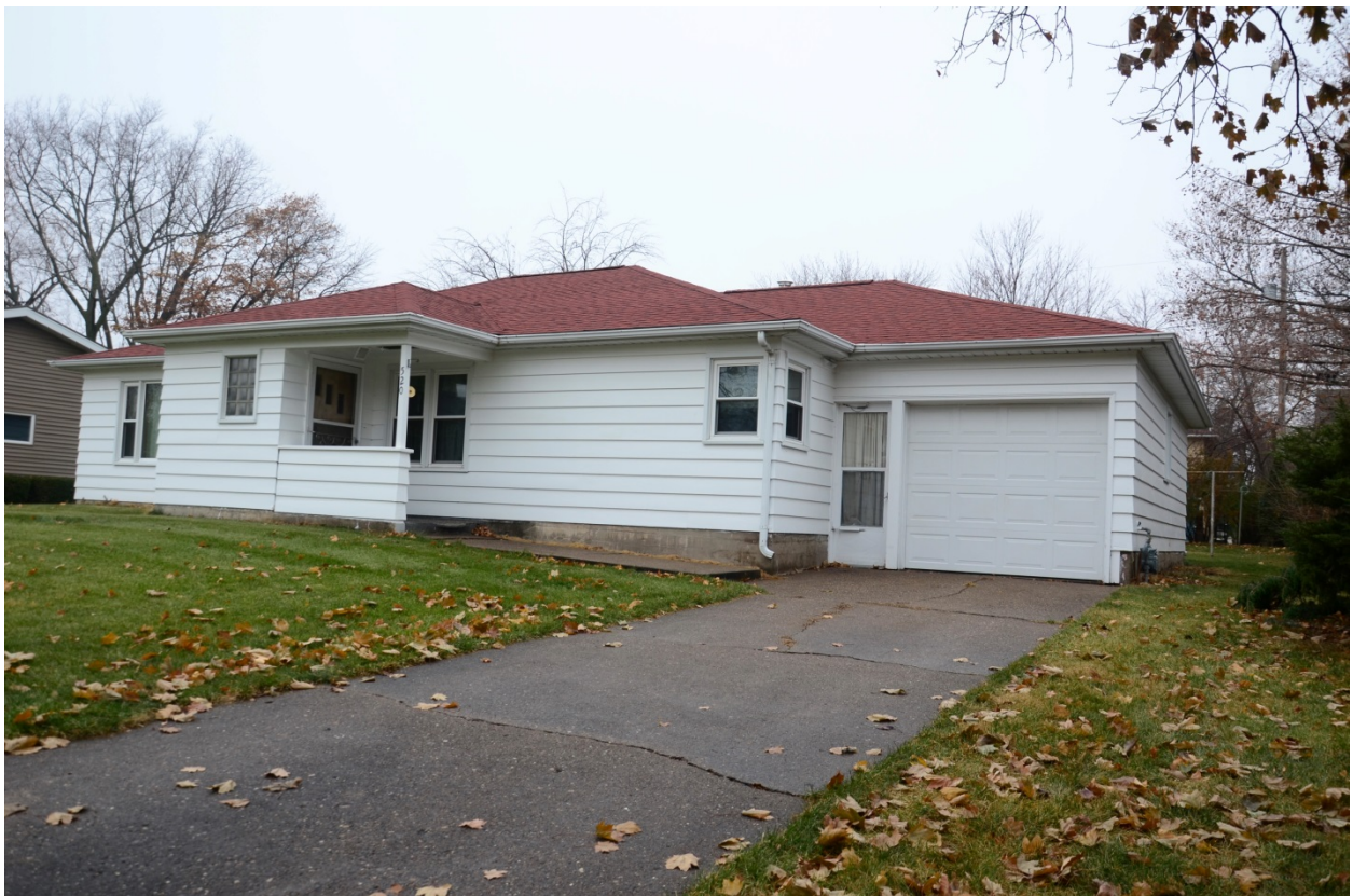
Figure 63. Howard and Anne Hess House at 520 W. Jefferson (December 2014)
