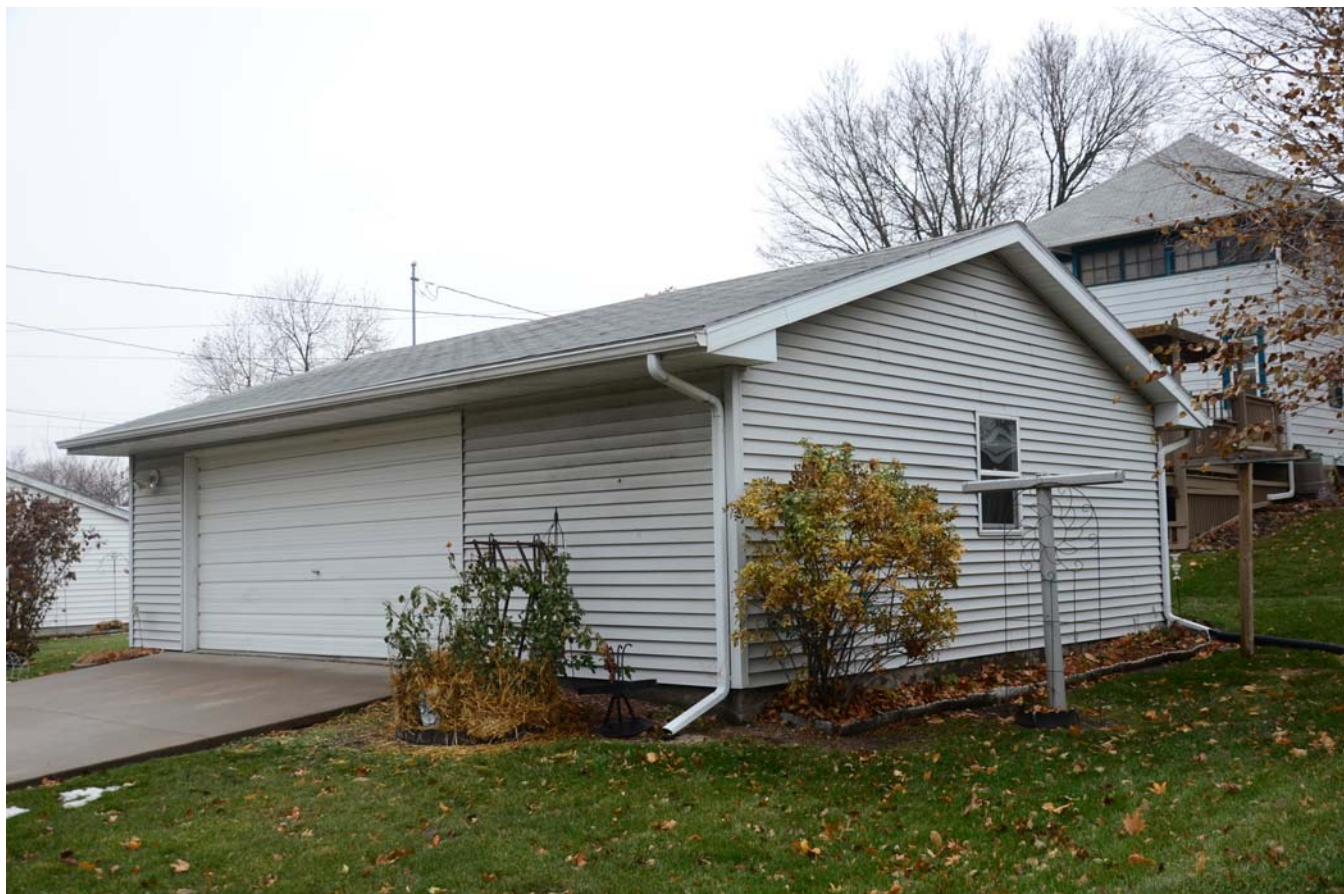
Photograph 92-00754-004 - Garage, looking northwest (December 2014)
