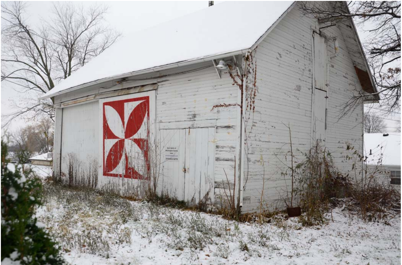
Photograph 92-00728-005 - Outbuilding, looking southwest (December 2014)
