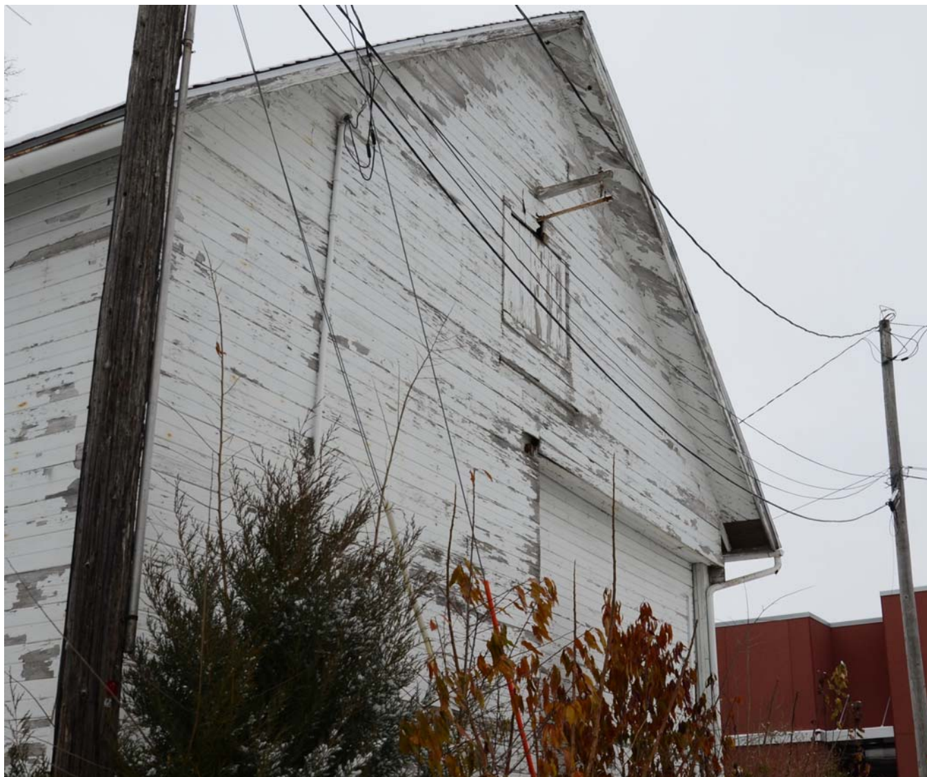
Photograph 92-00728-006 - Outbuilding, looking northeast (December 2014)
