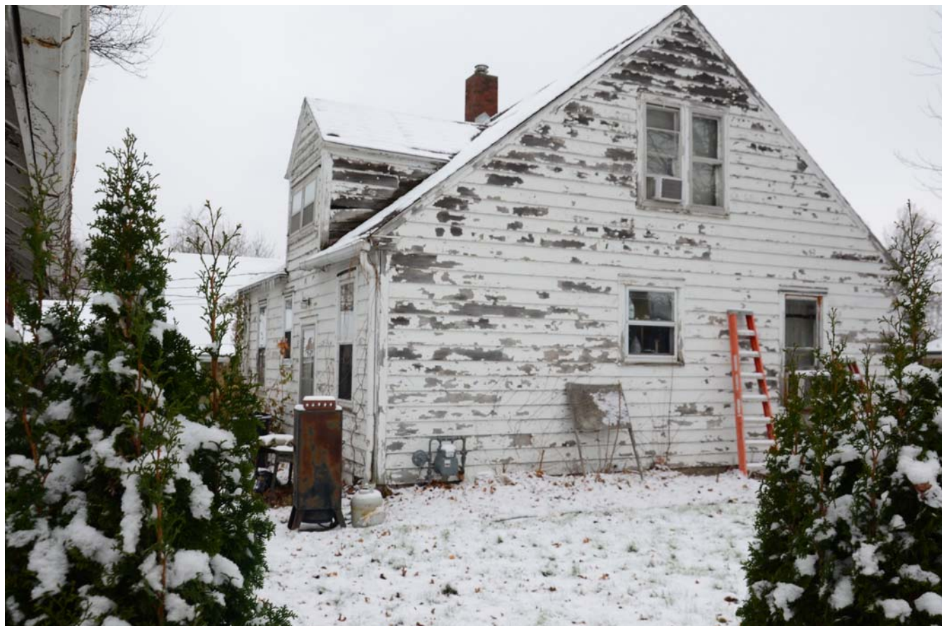
Photograph 92-00728-002 - House, looking west (December 2014)
