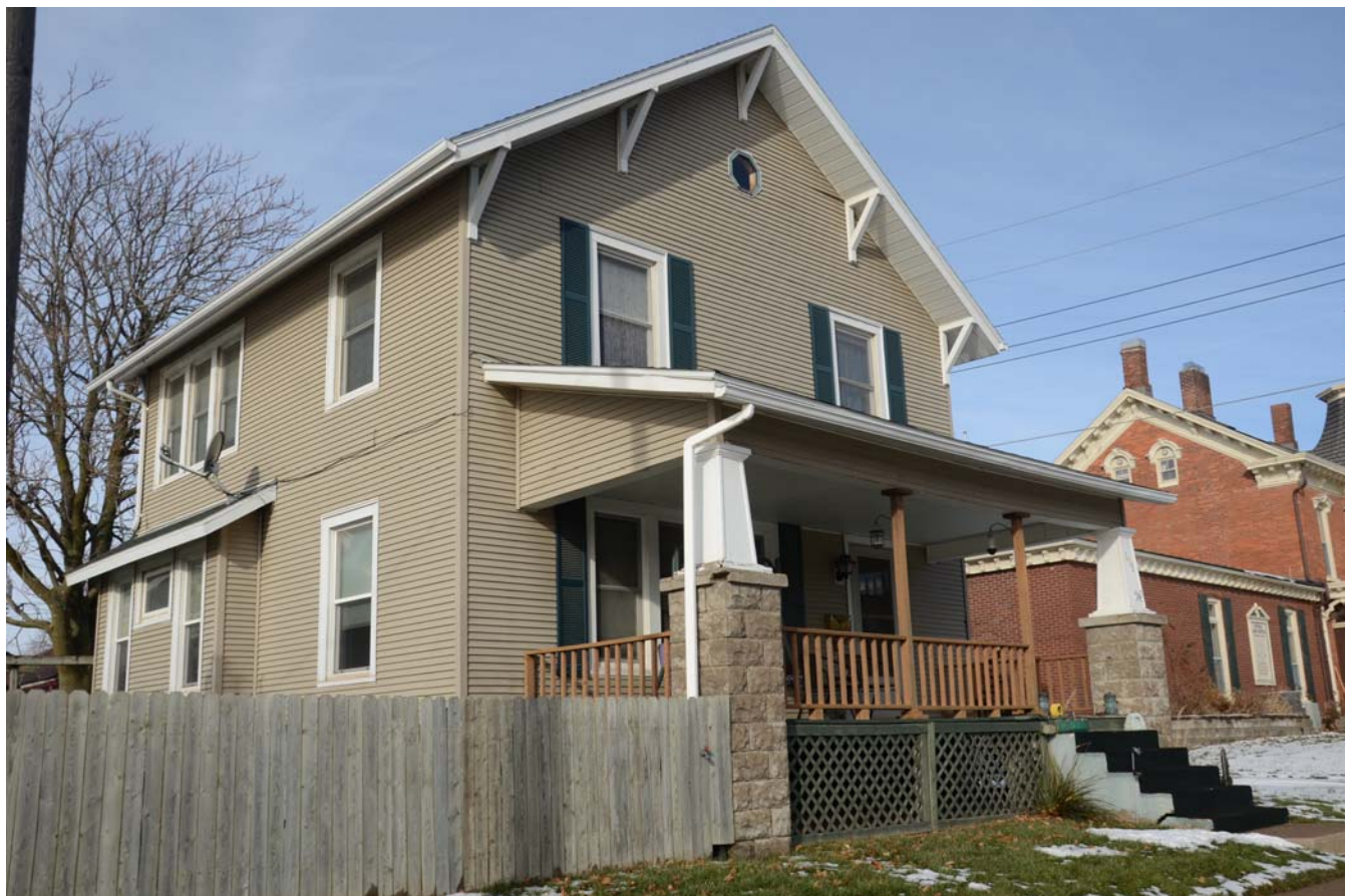
Photograph 92-00757-002 - House, looking northwest (December 2014)
