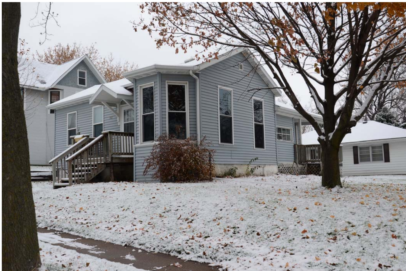
Photograph 92-00459-002 - House, looking southeast (December 2014)
