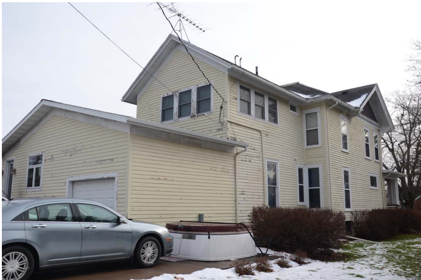
Photograph 92-00383-003 - House, looking southeast (December 2014)
