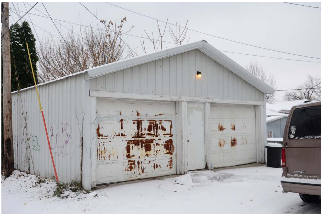
Photograph 92-00159-004 - Garage, looking southeast (December 2014)
