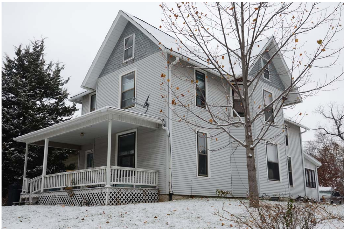
Photograph 92-00159-002 - House, looking northwest (December 2014)
