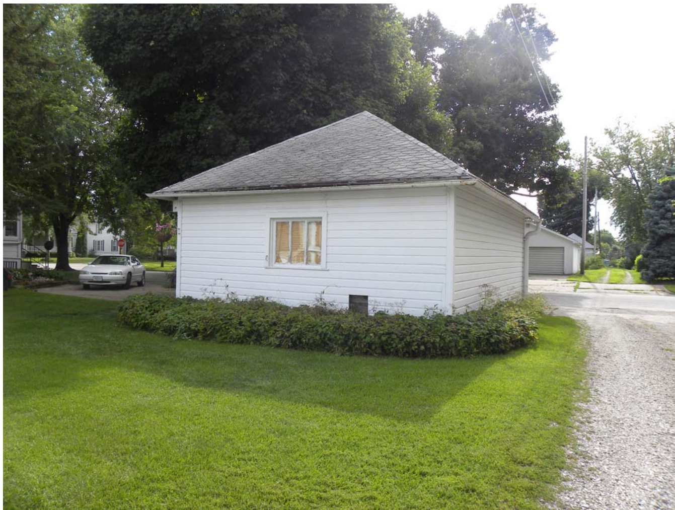
Photograph 92-00384-005 - Garage, looking west (July 2015)
