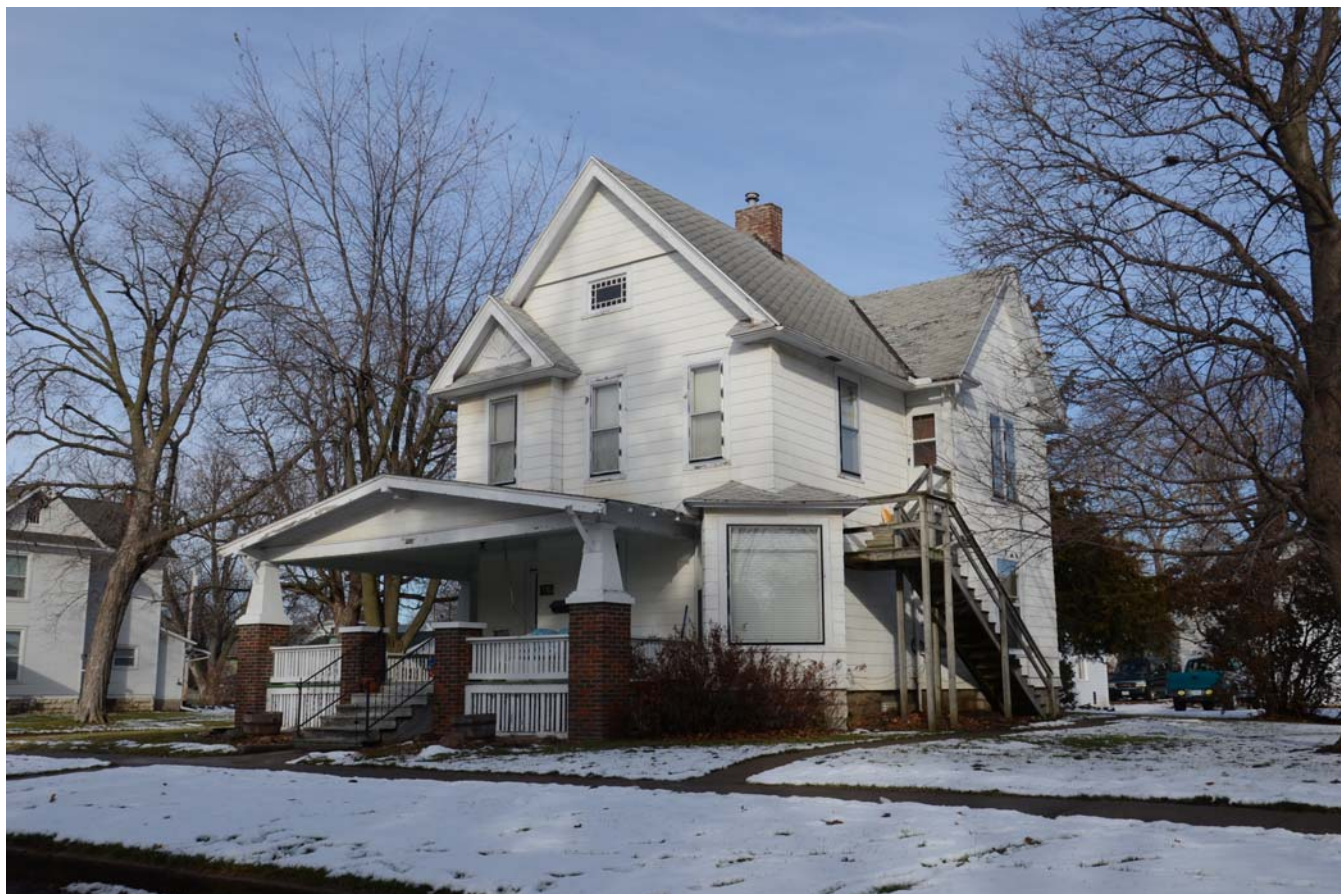
Photograph 92-00384-002 - House, looking northwest (December 2014)
