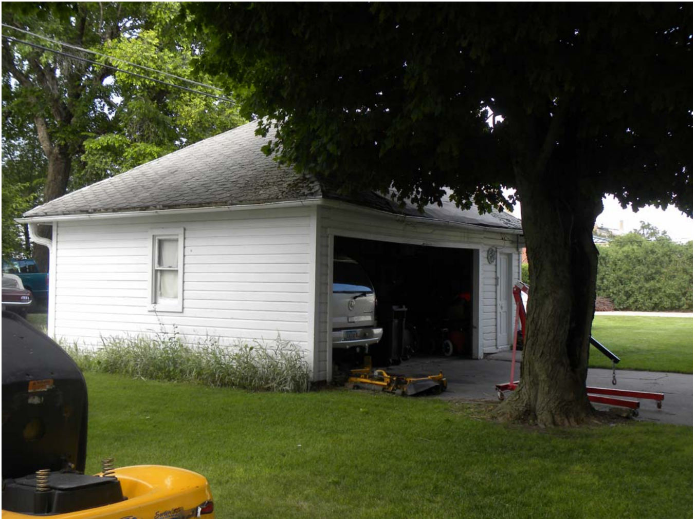
Photograph 92-00384-004 - Garage, looking northeast (July 2015)
