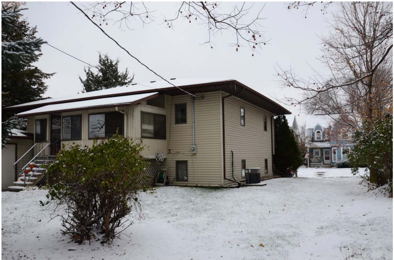
Photograph 92-00731-002 - House, looking southeast (December 2014)
