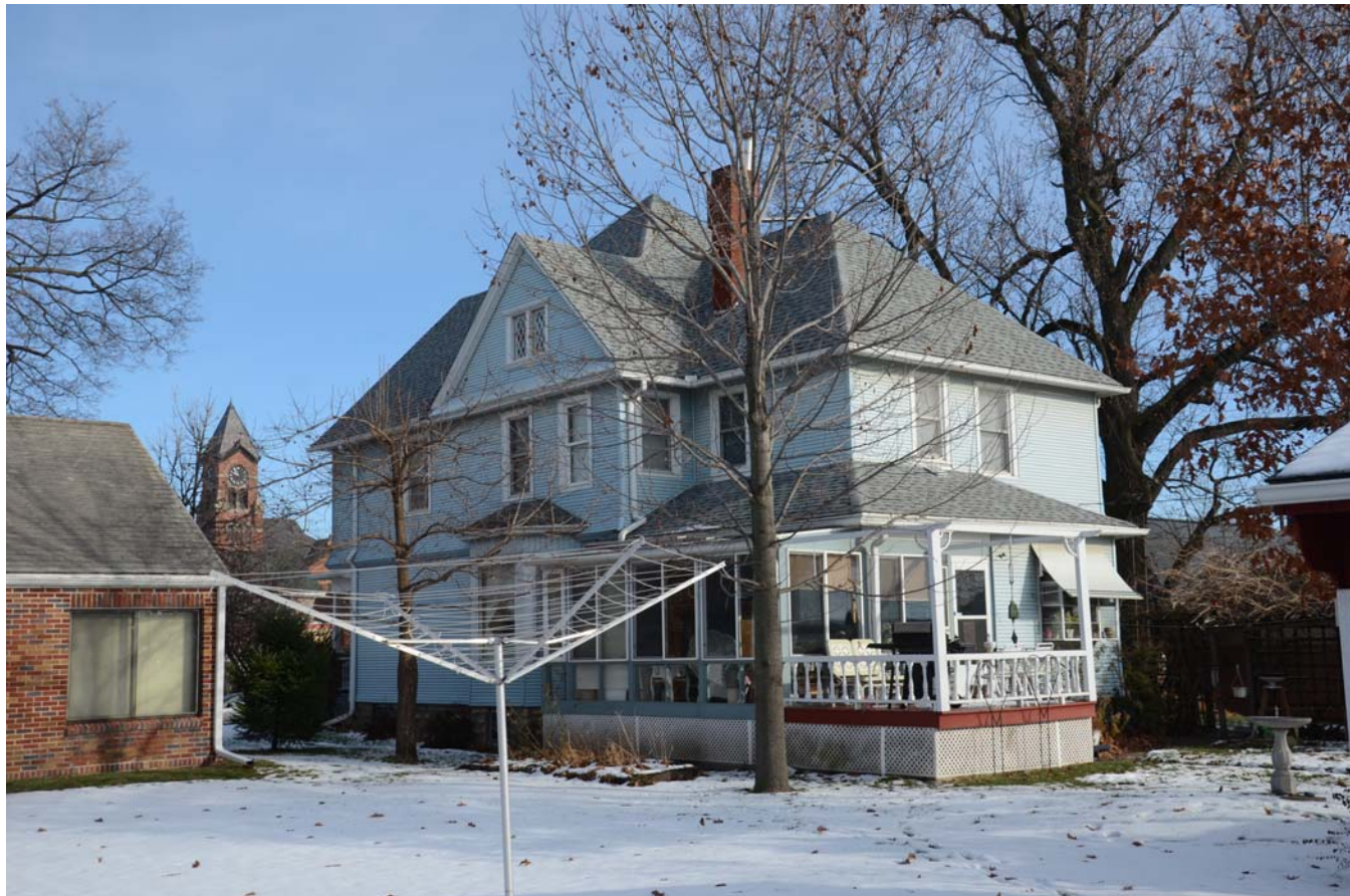
Photograph 92-00367-004 - House, looking northeast (December 2014)
