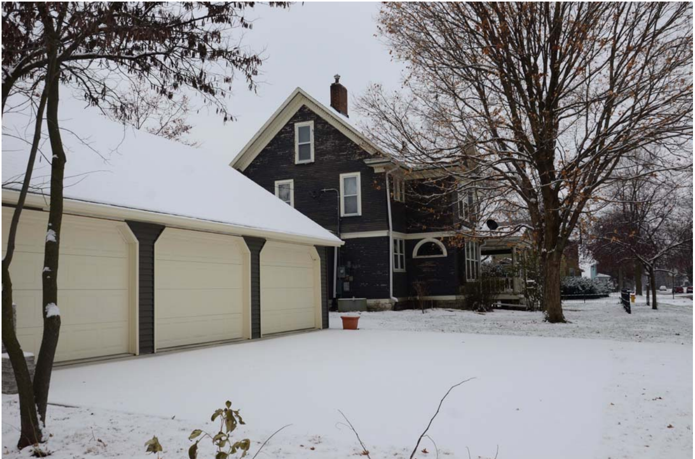
Photograph 92-00424-007 - Garage, looking southeast (December 2014)
