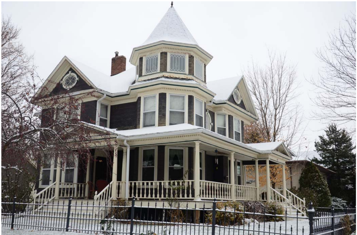
Photograph 92-00424-002 - House, looking northeast (December 2014)
