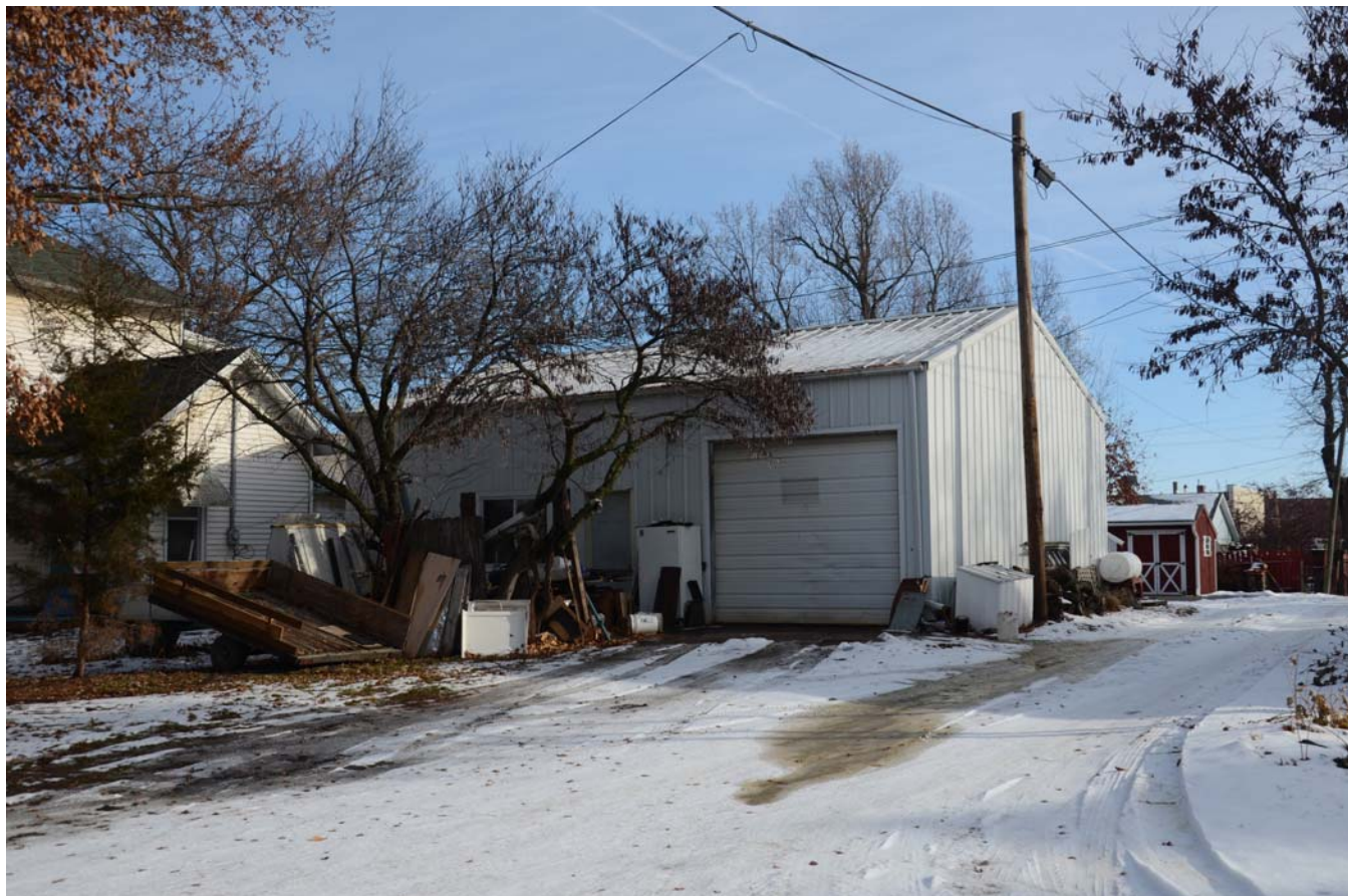
Photograph 92-00368-004 - Garage, looking northeast (December 2014)
