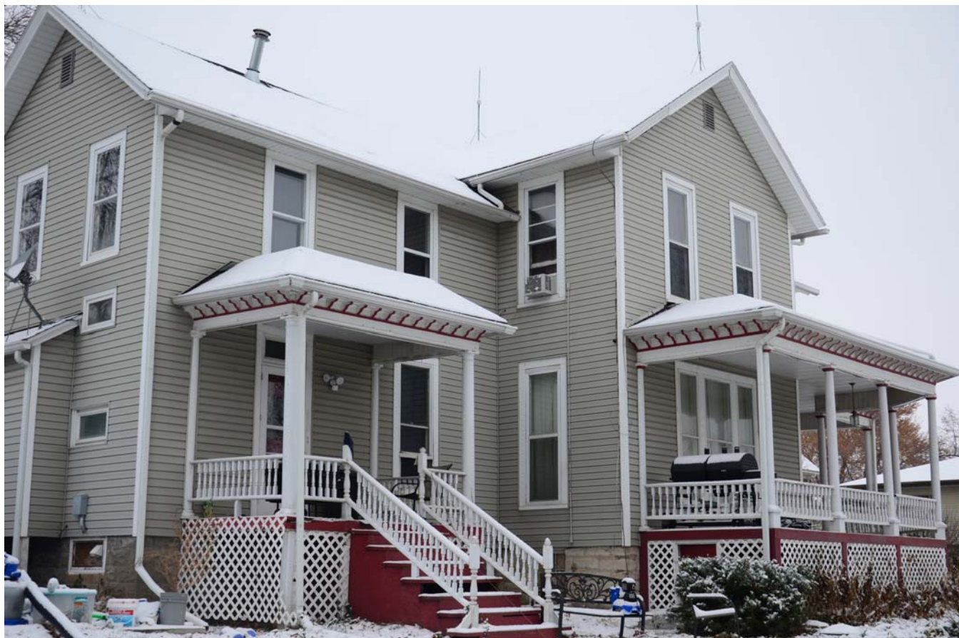
Photograph 92-00420-003 - House, looking northwest (December 2014)
