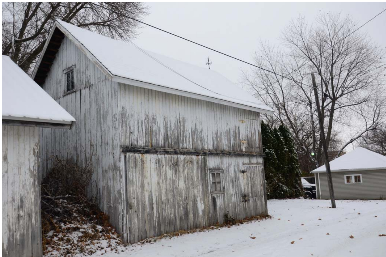
Photograph 92-00421-004 - Garage, looking northeast (December 2014)
