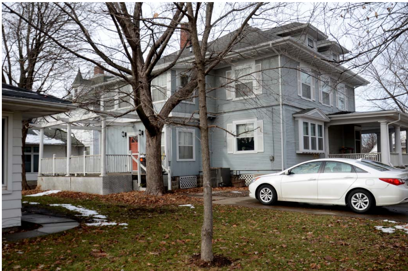
Photograph 92-00369-003 - House, looking northwest (December 2014)
