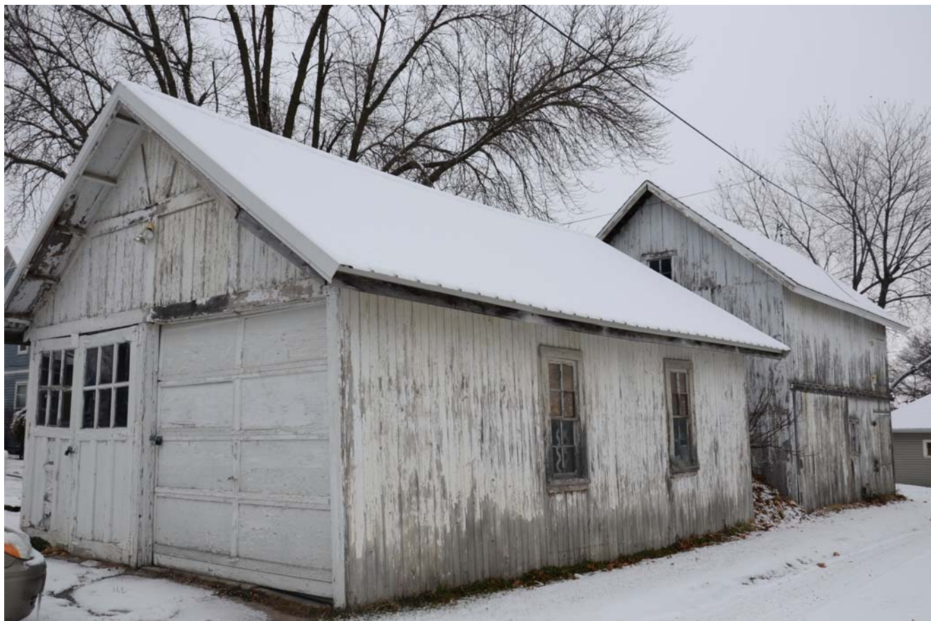
Photograph 92-00733-005 - Garage, looking northeast (December 2014)
