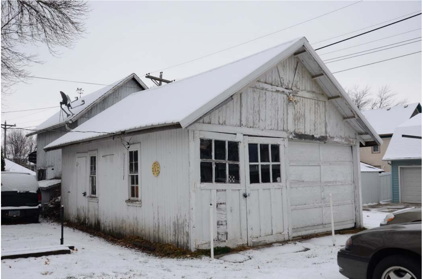
Photograph 92-00733-004 - Garage, looking southeast (December 2014)
