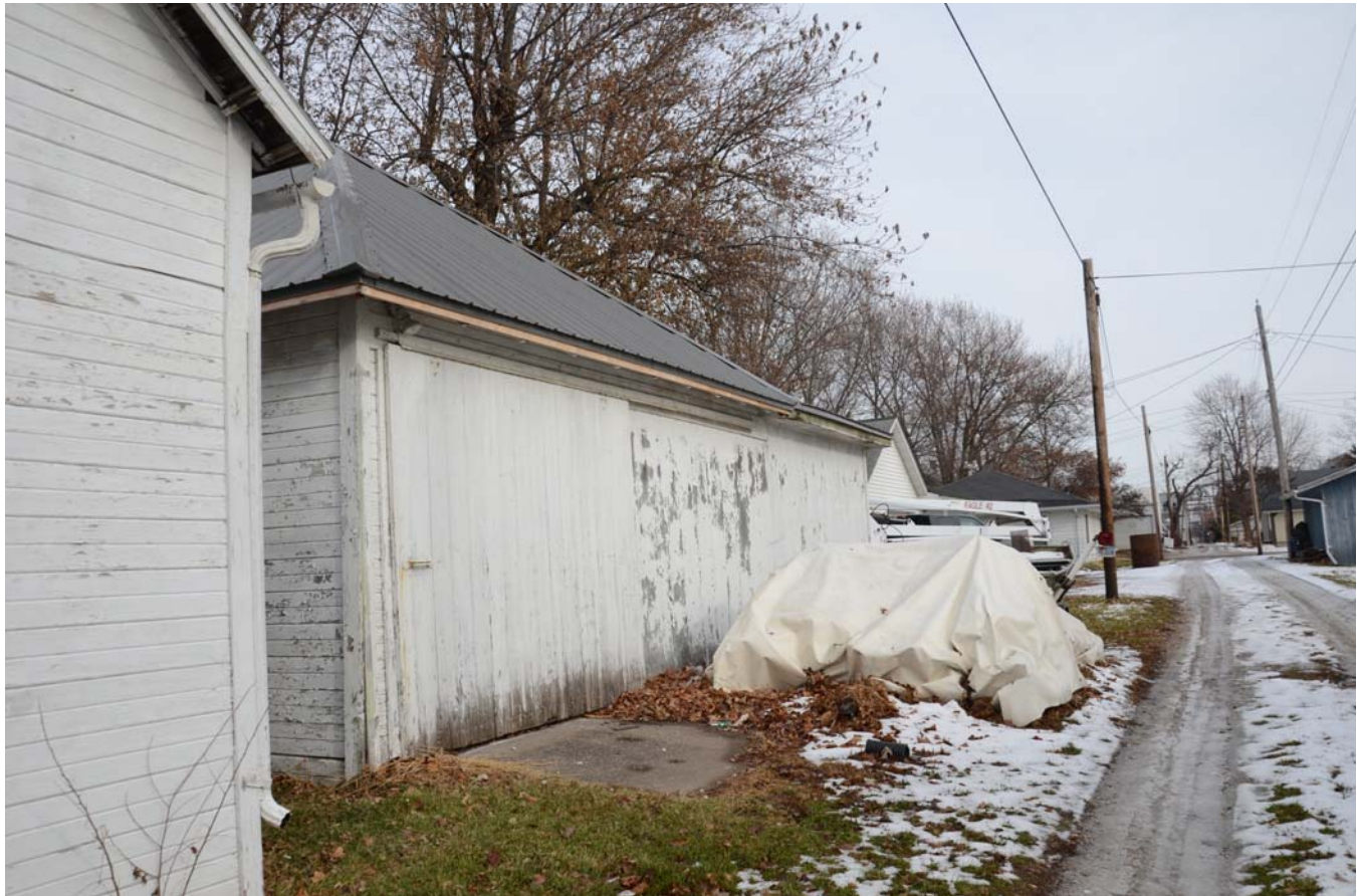
Photograph 92-00371-004 - Garage, looking northeast (December 2014)
