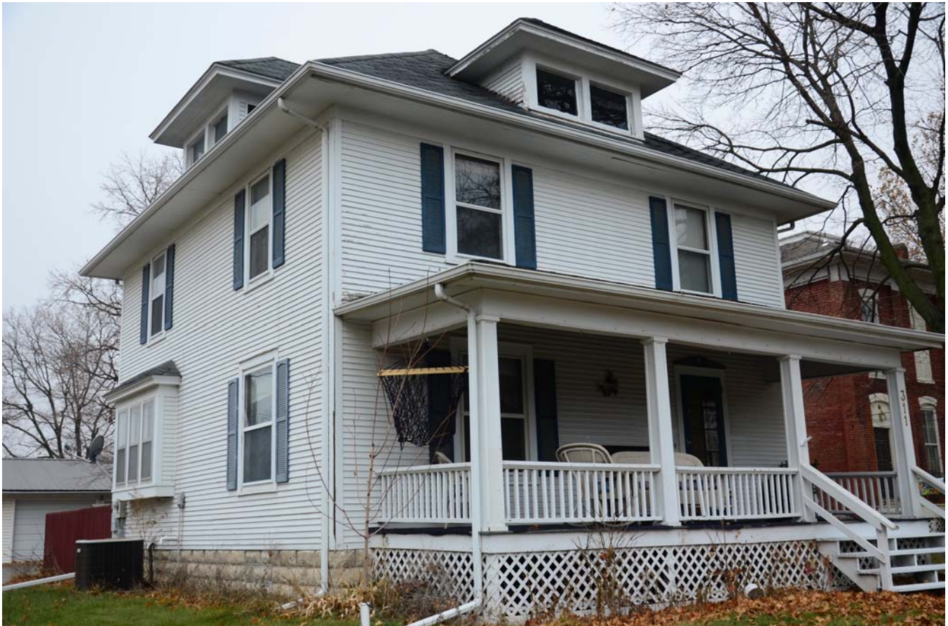
Photograph 92-00427-002 - House, looking northwest (December 2014)
