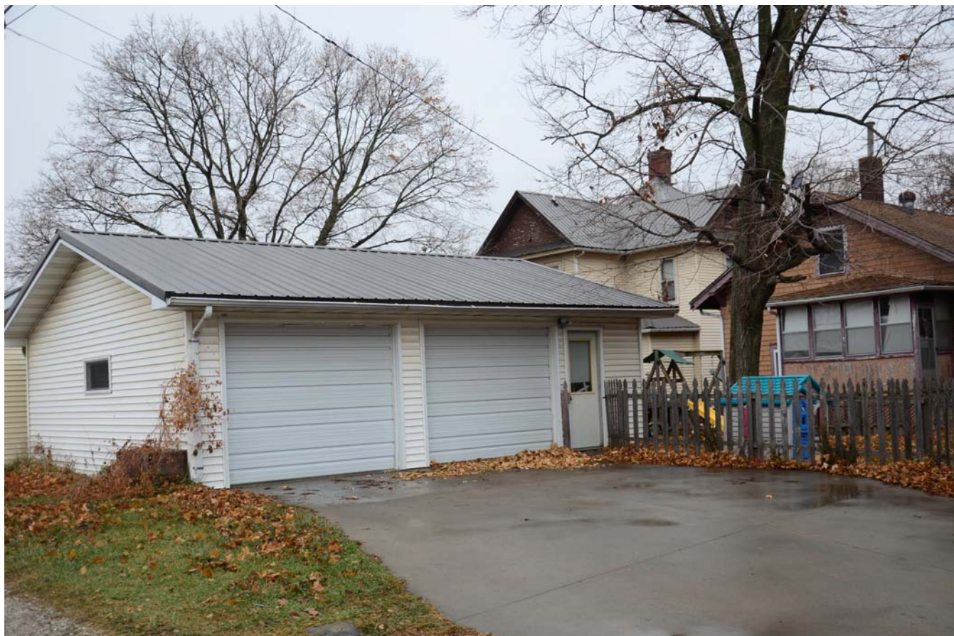
Photograph 92-00427-004 - Garage, looking northwest (December 2014)
