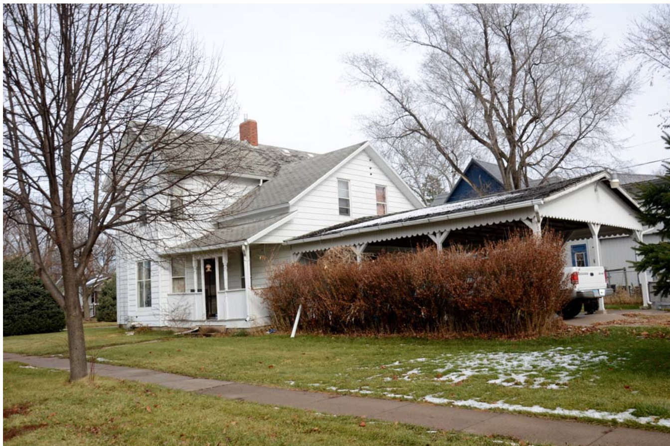
Photograph 92-00372-003 - House, looking northeast (December 2014)
