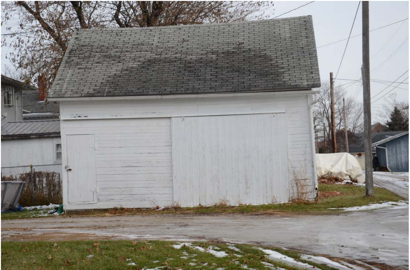
Photograph 92-00372-004 - Garage, looking east (December 2014)
