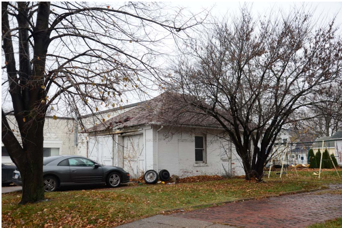
Photograph 92-00429-005 - Garage, looking northwest (December 2014)
