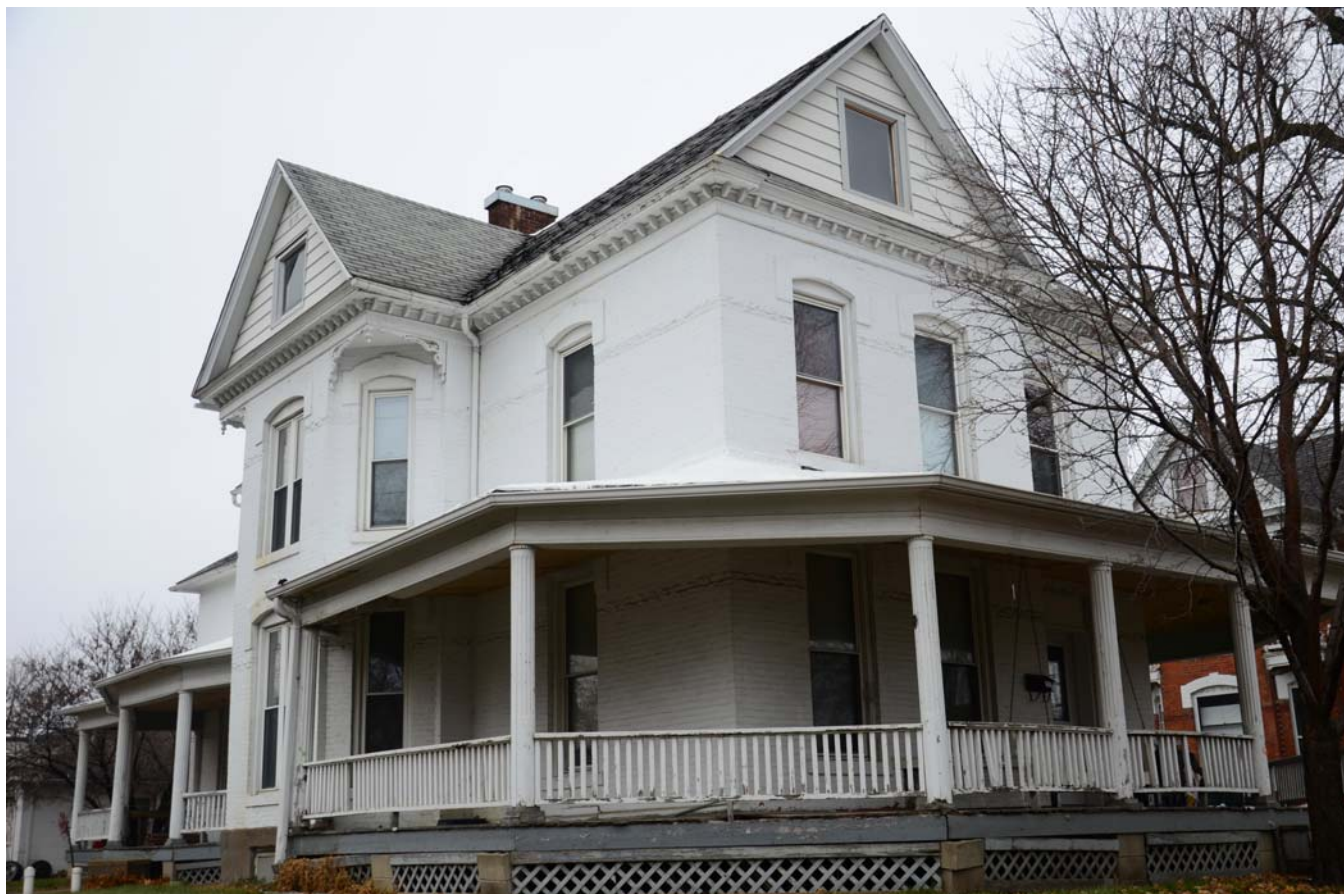
Photograph 92-00429-002 - House, looking northwest (December 2014)
