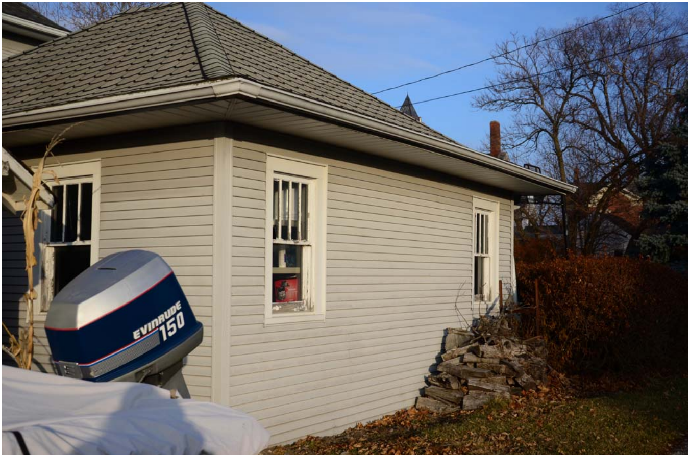
Photograph 92-00400-005 - Garage, looking northeast (December 2014)
