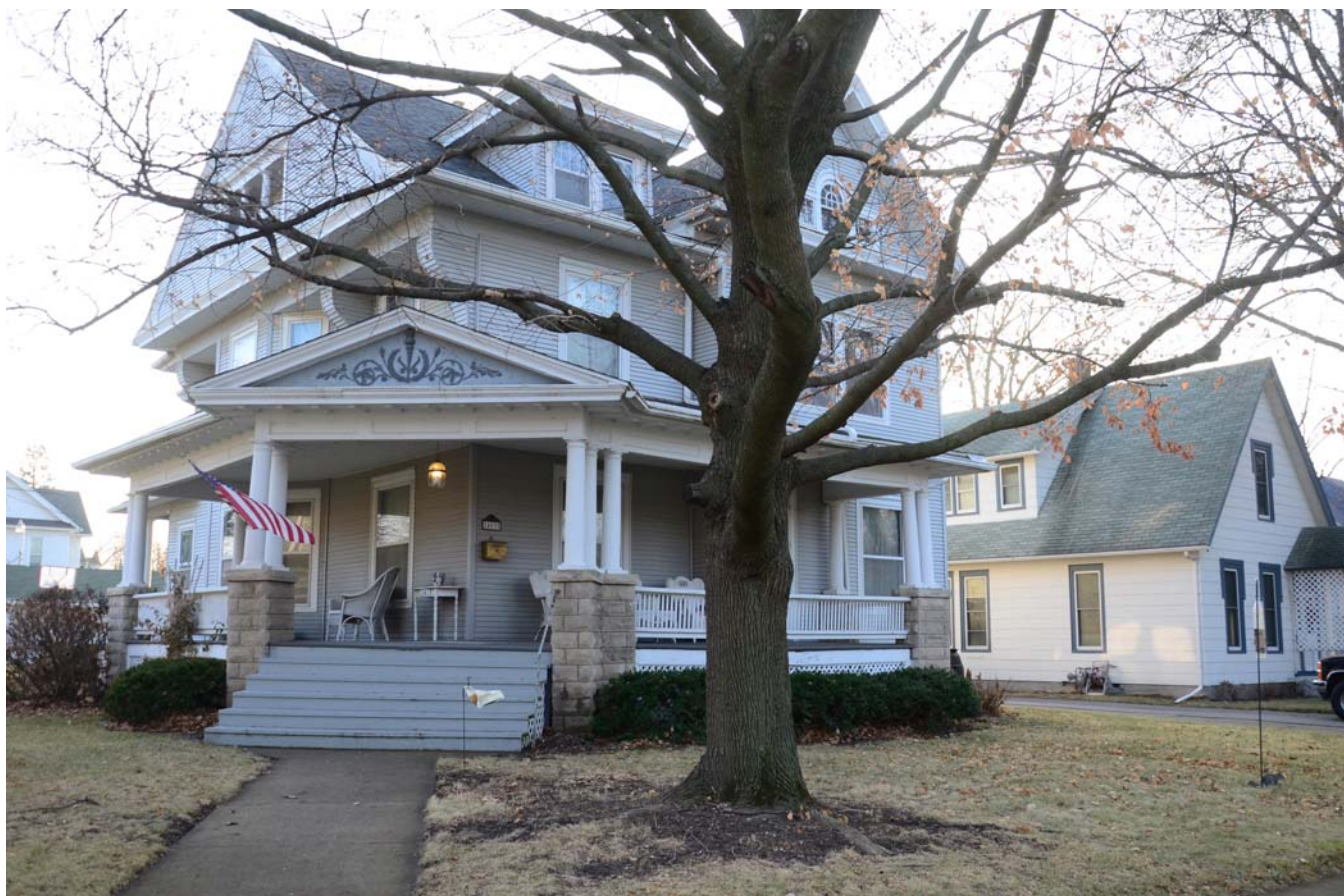
Photograph 92-00400-001 - East and north (front) elevations, looking southwest (December 2014)
