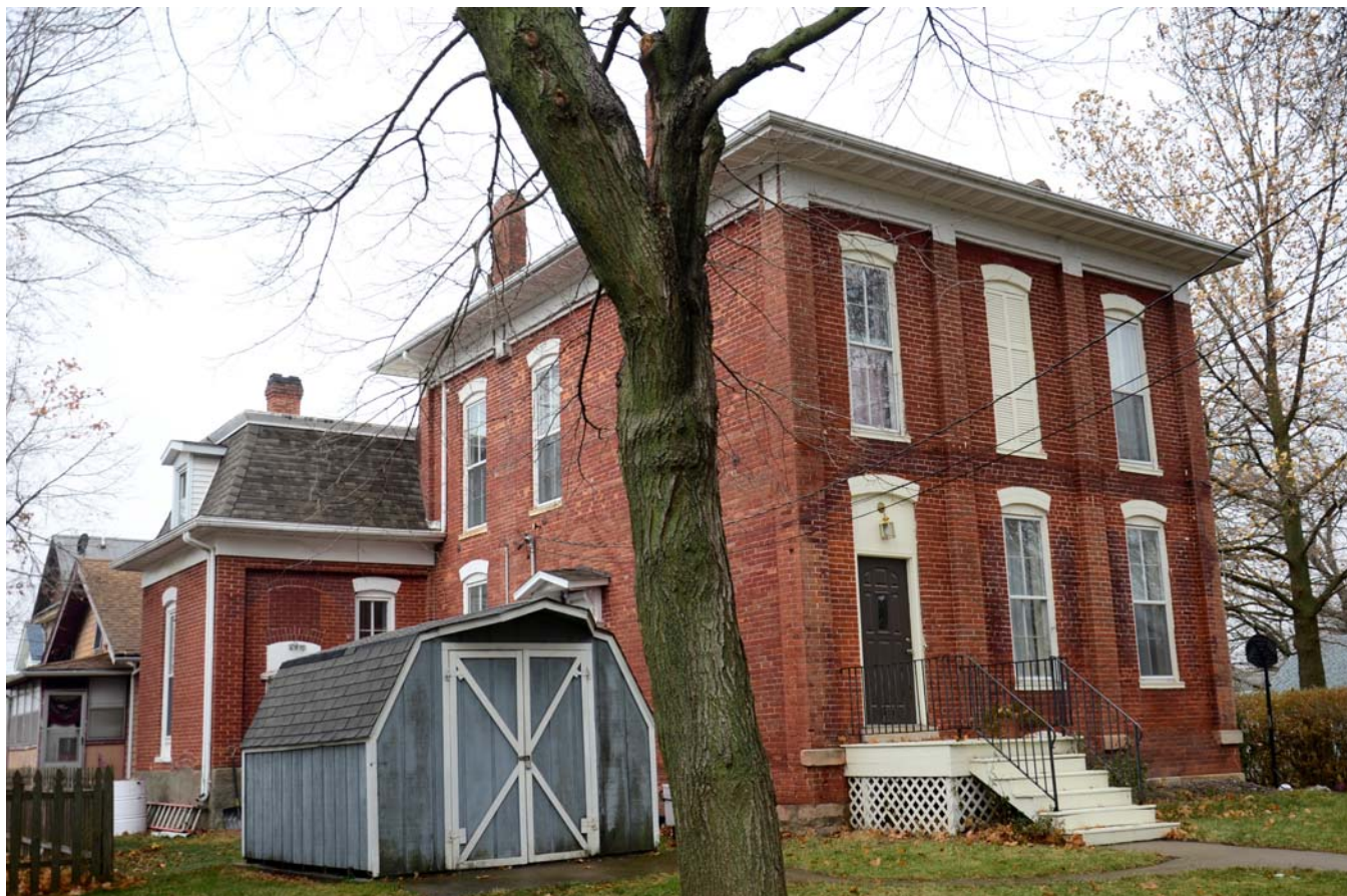
Photograph 92-00155-002 - House, looking northwest (December 2014)
