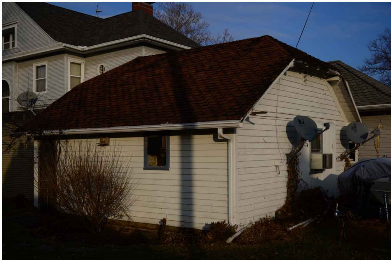
Photograph 92-00401-004 - Garage, looking northeast (December 2014)
