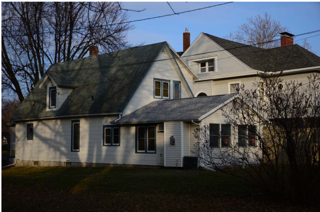
Photograph 92-00401-003 - West and rear (south) elevations, looking northeast (December 2014)
