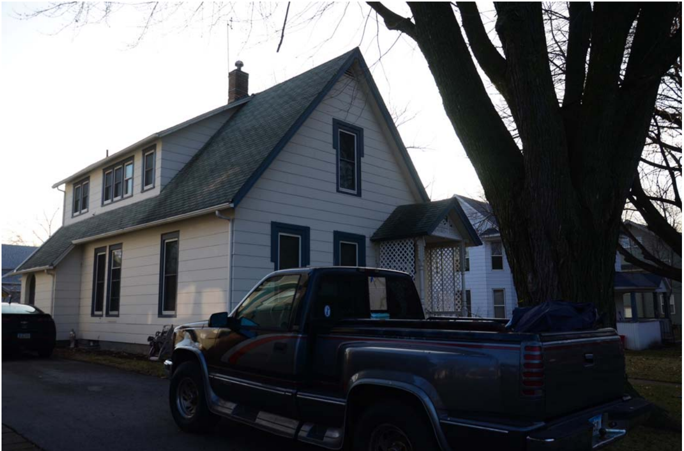
Photograph 92-00401-002 - North (front) and east elevations, looking southwest (December 2014)
