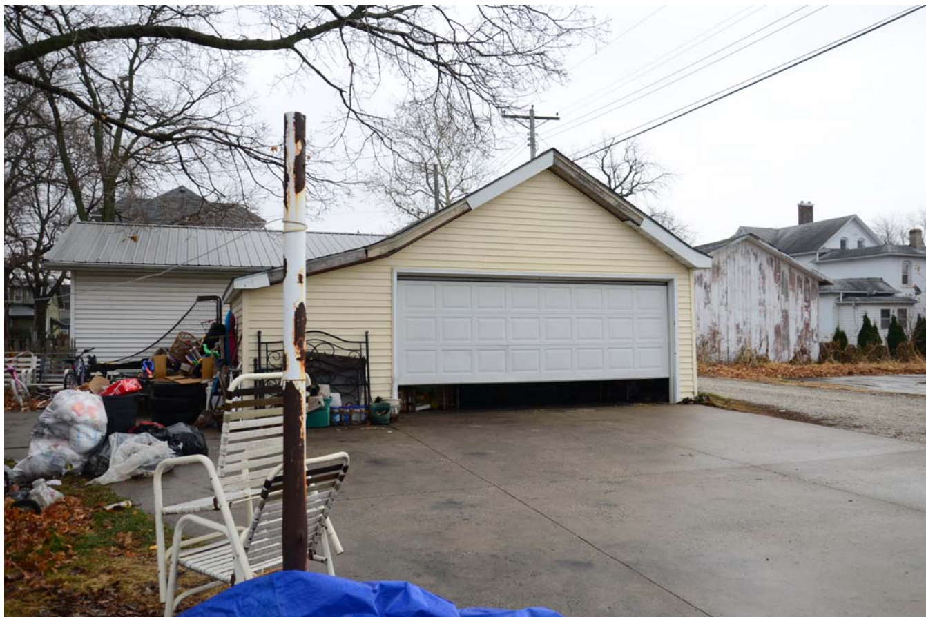
Photograph 92-00423-004 - Garage, looking southeast (December 2014)
