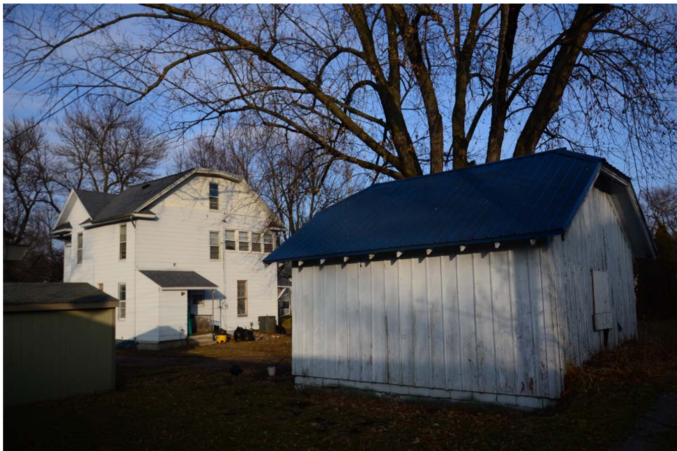
Photograph 92-00163-004 - Garage, looking northeast (December 2014)
