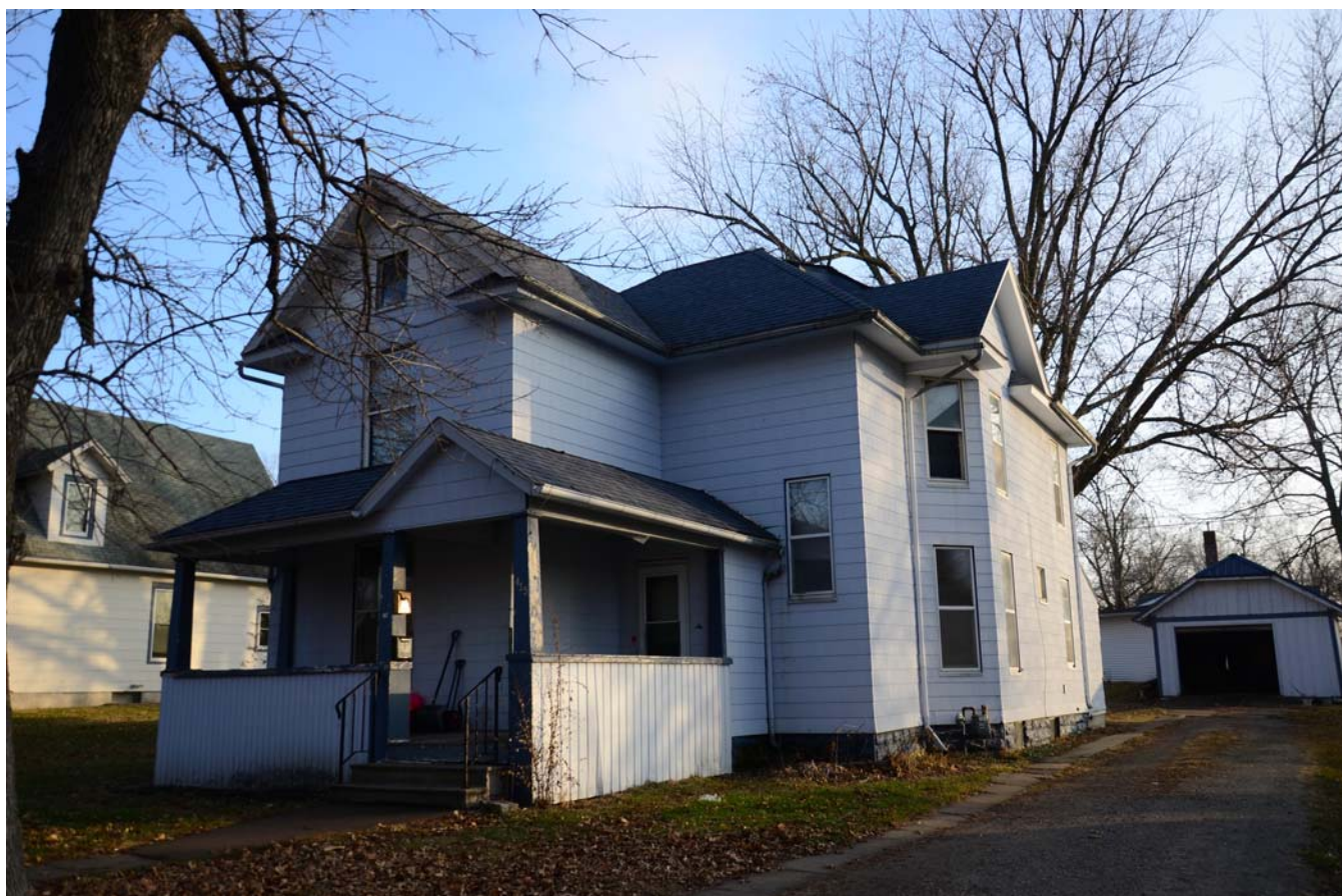
Photograph 92-00163-001 - House and garage, looking southeast (December 2014)
