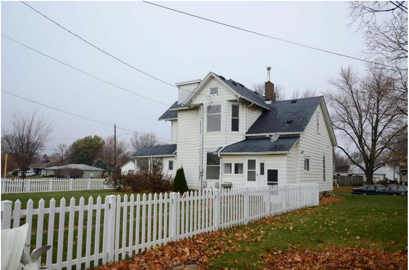
Photograph 92-00430-003 - House, looking northwest (December 2014)
