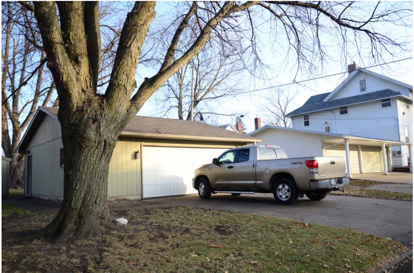
Photograph 92-00403-004 - Garage, looking southeast (December 2014)
