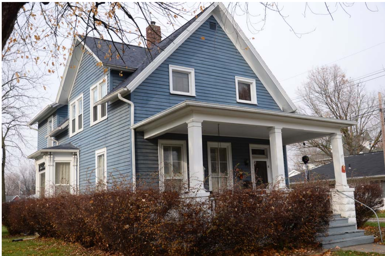
Photograph 92-00734-002 - House, looking northwest (December 2014)
