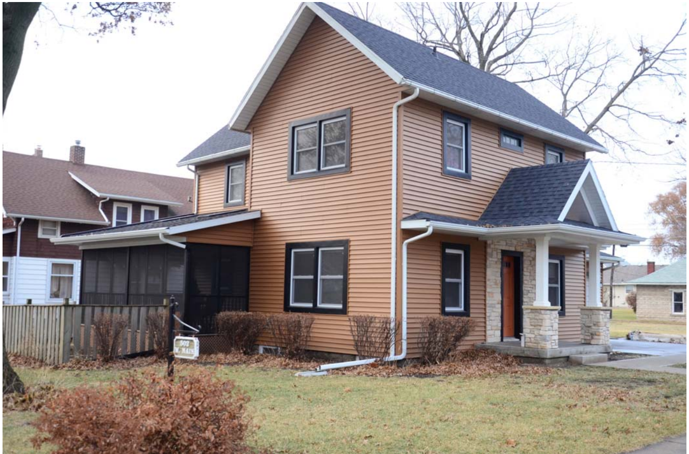
Photograph 92-00775-001 - House, looking northwest (December 2014)
