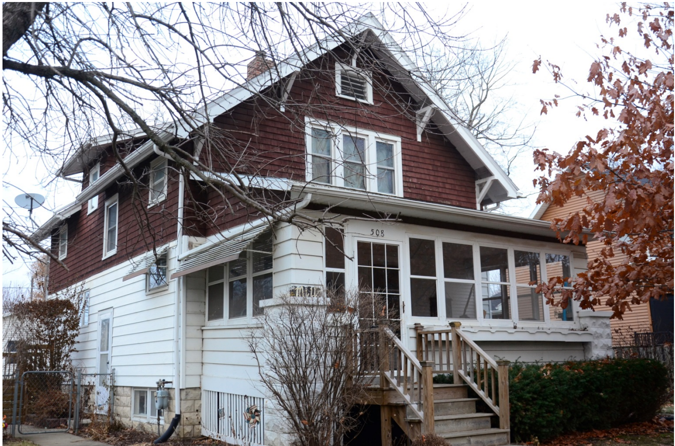
Photograph 92-00416-001 - House, looking northeast (December 2014)
