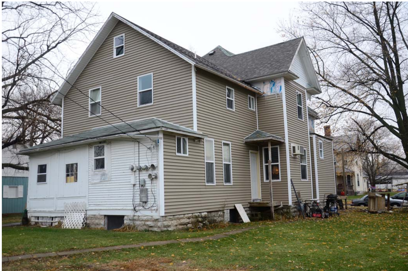
Photograph 92-00735-003 - House, looking southeast (December 2014)
