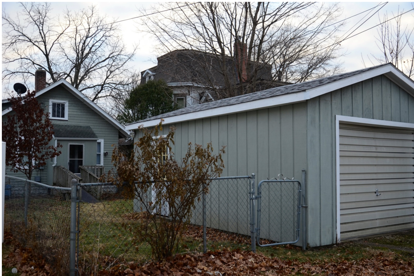
Photograph 92-00776-004 - Garage, looking southwest (December 2014)
