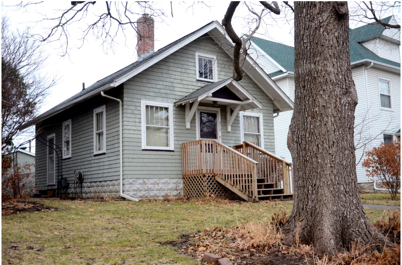
Photograph 92-00776-001 - House, looking northeast (December 2014)
