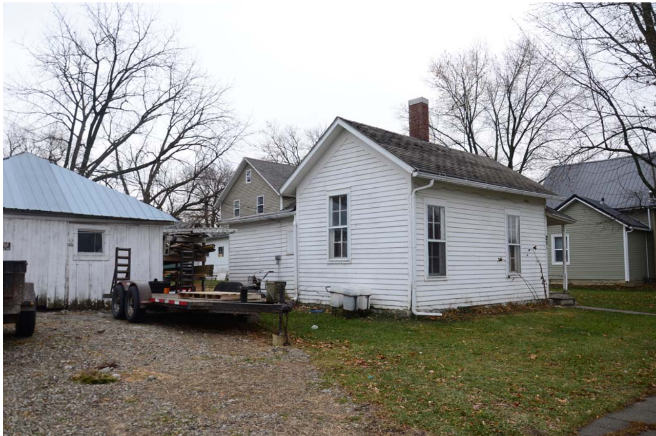
Photograph 92-00737-002 - House, looking southeast (December 2014)
