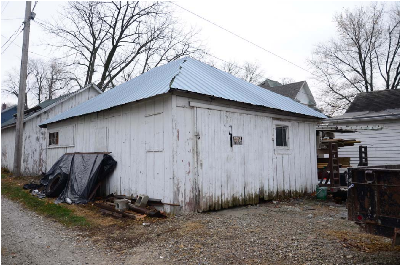
Photograph 92-00737-005 - Garage, looking southeast (December 2014)
