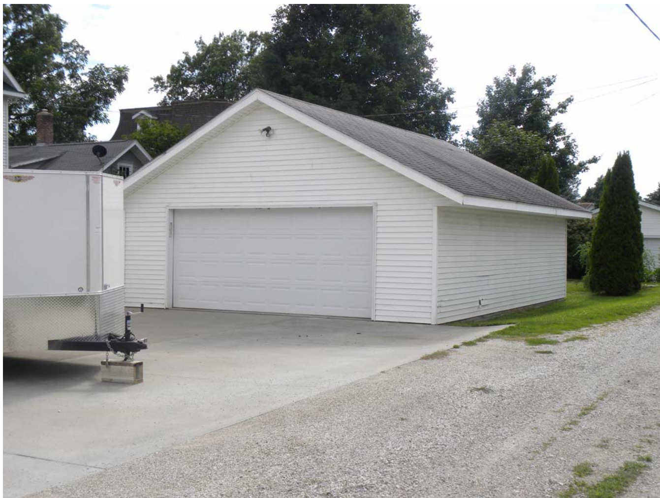
Photograph 92-00417-003 - Garage, looking southwest (July 2015)
