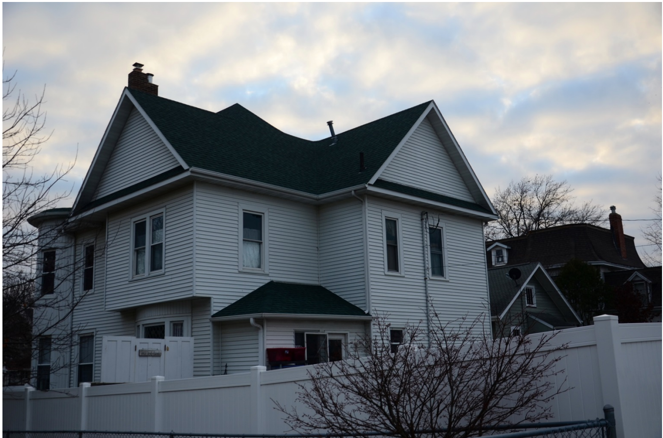
Photograph 92-00417-002 - House, looking southwest (December 2014)
