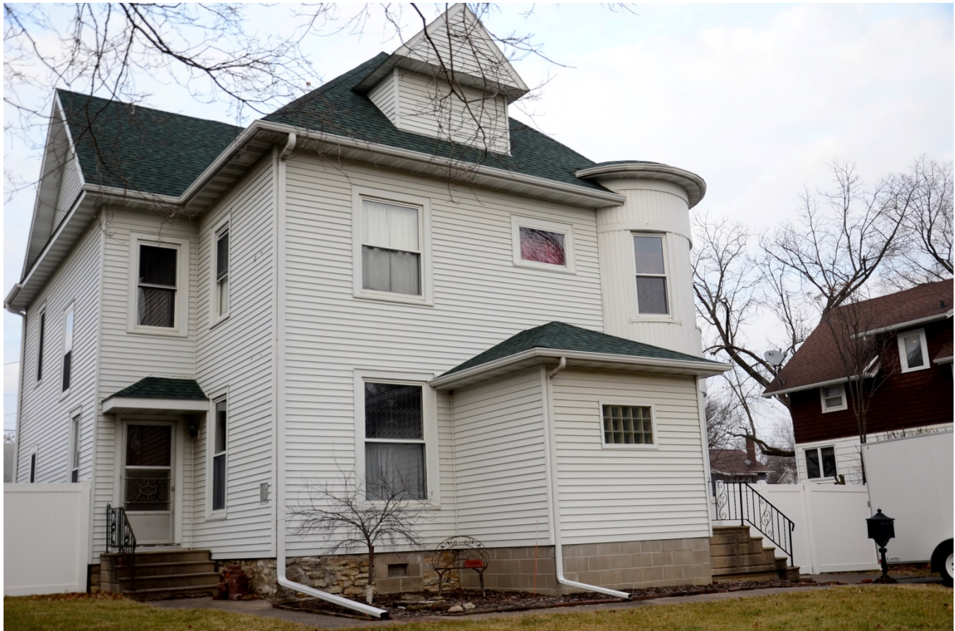
Photograph 92-00417-001 - House, looking northeast (December 2014)
