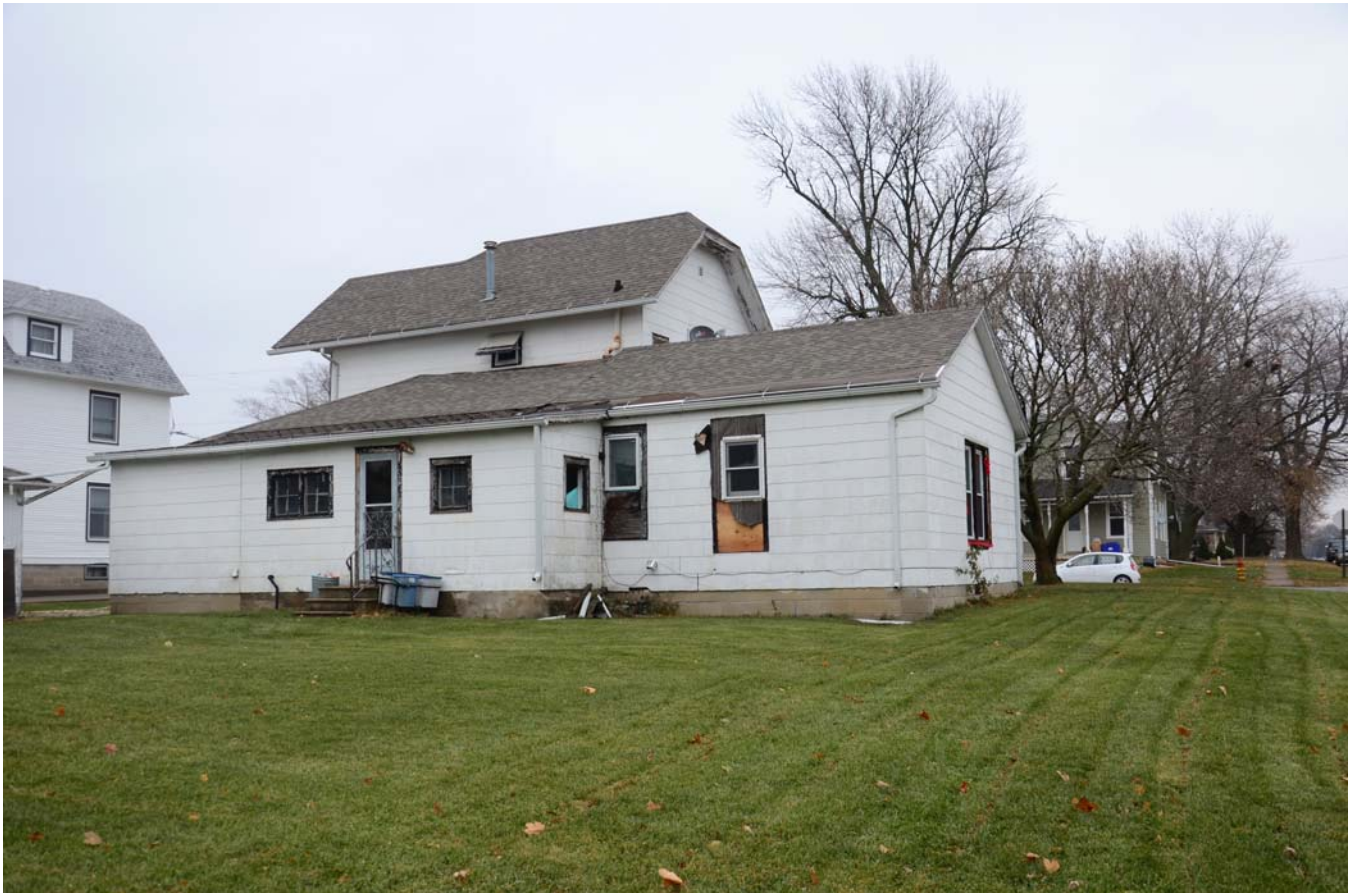
Photograph 92-00739-003 - House, looking northeast (December 2014)
