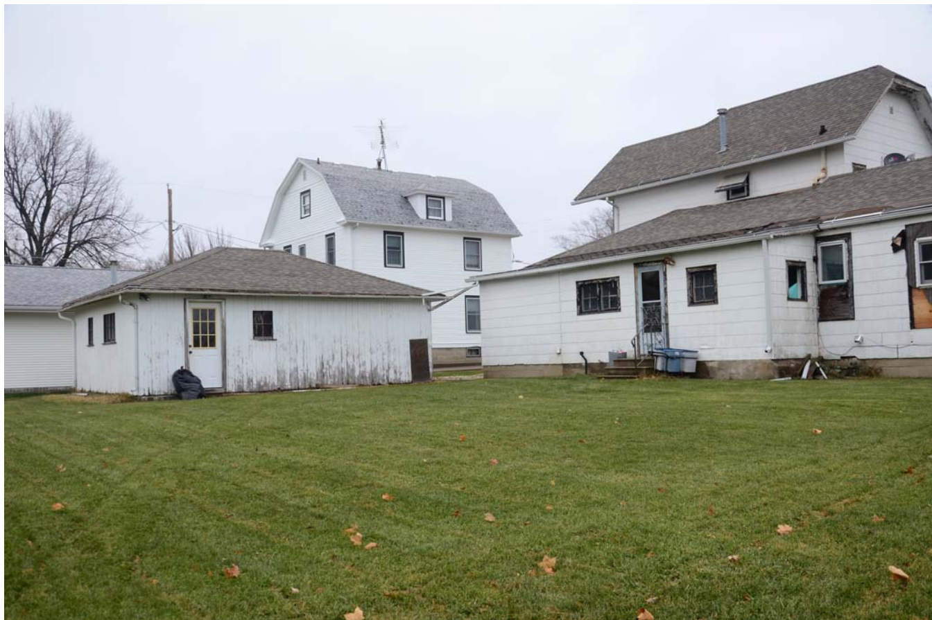
Photograph 92-00739-004 - Garage and house, looking northeast (December 2014)
