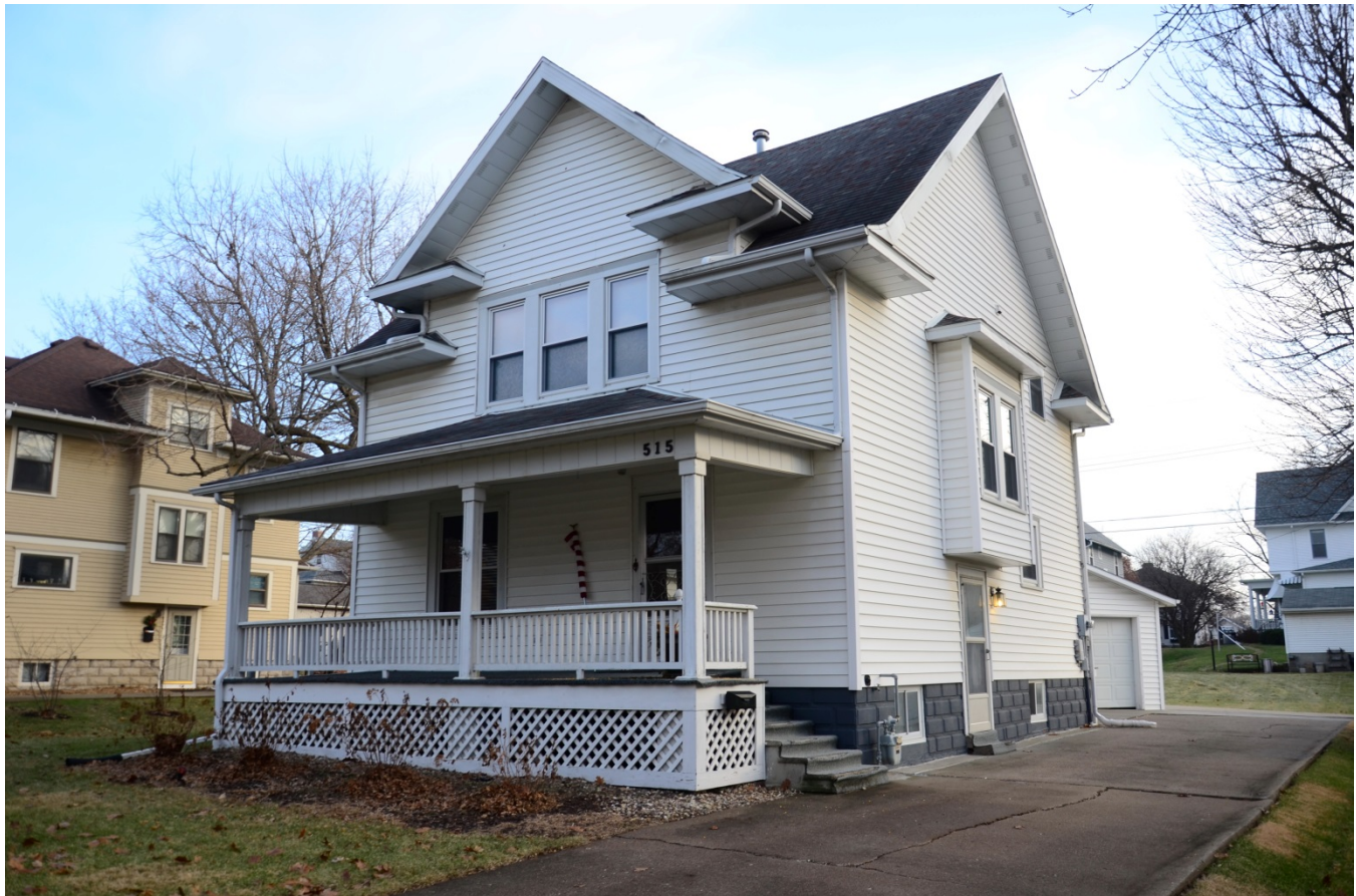
Photograph 92-00406-001 - House, looking southeast (December 2014)
