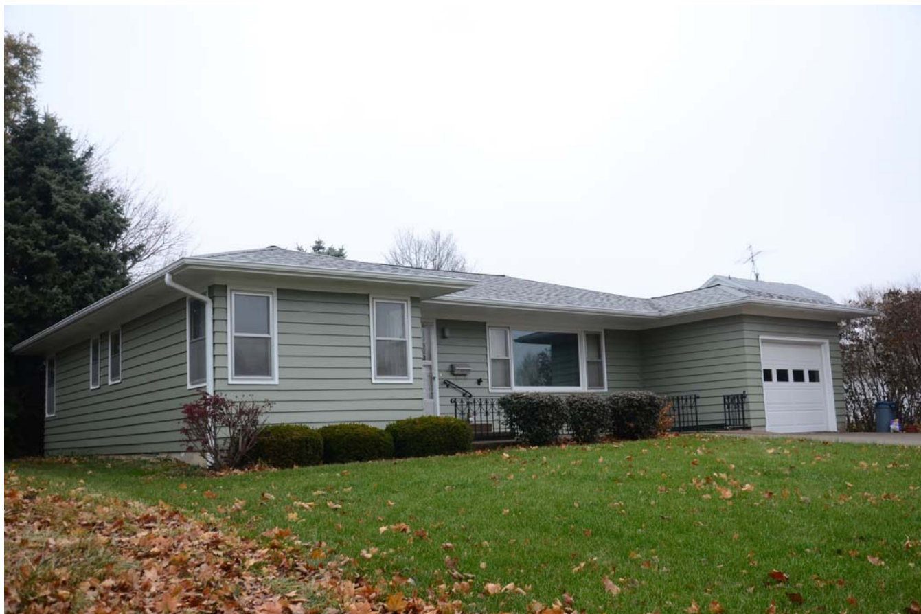
Photograph 92-00740-001 - House, looking northeast (December 2014)
