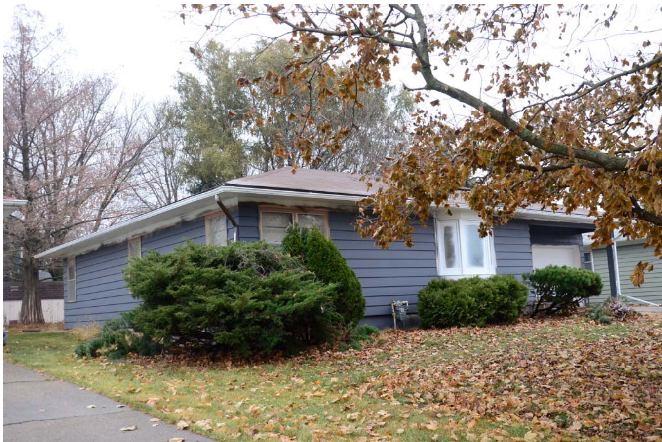
Photograph 92-00741-001 - House, looking northeast (December 2014)
