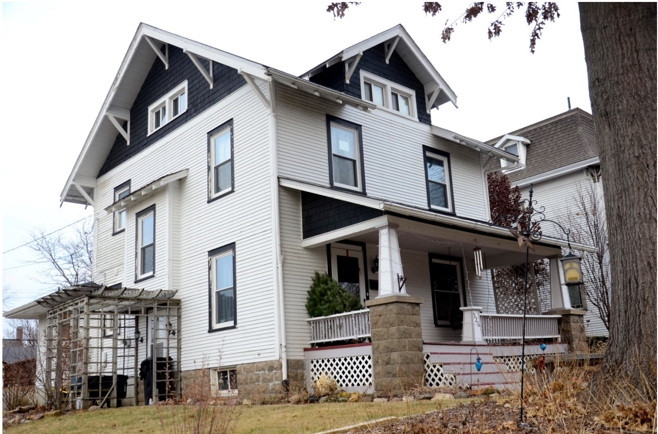
Photograph 92-00419-002 - House, looking northeast (December 2014)
