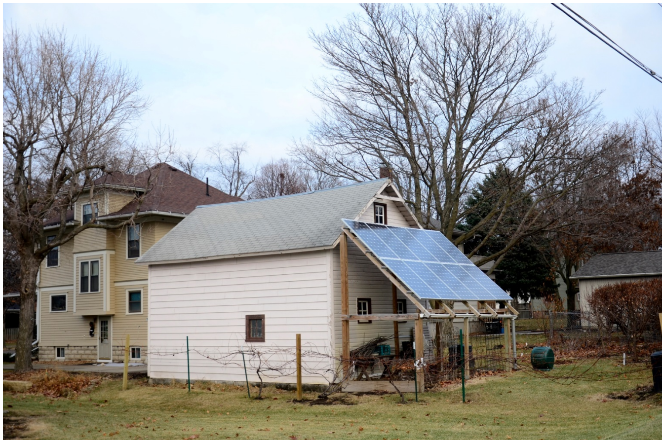
Photograph 92-00405-004 - Garage, looking northeast (December 2014)
