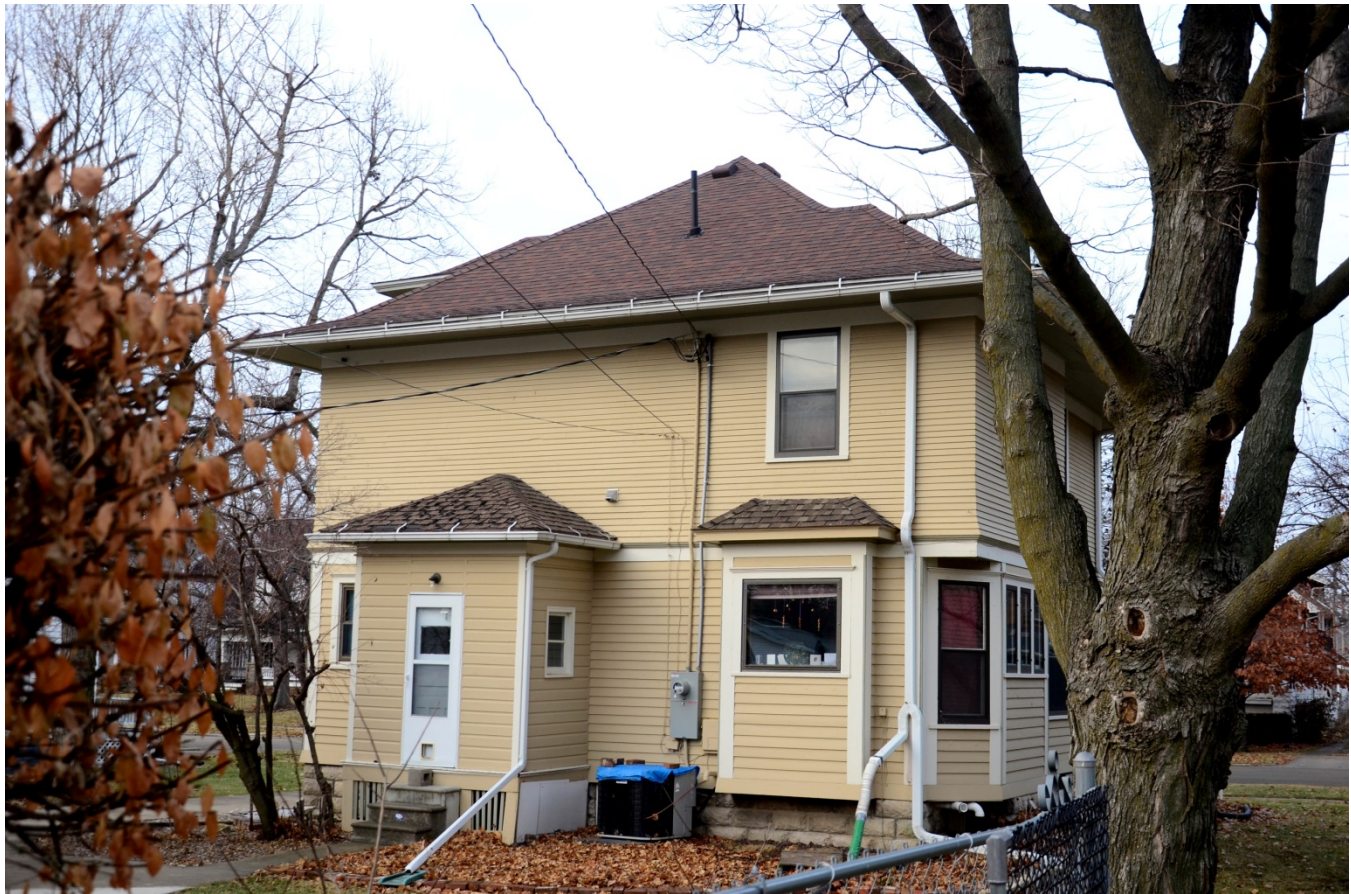
Photograph 92-00405-003 - House, looking north (December 2014)
