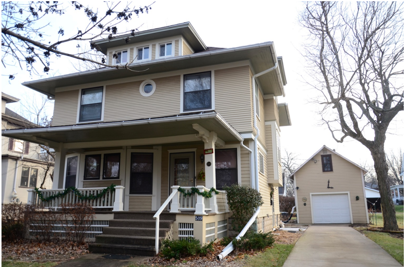
Photograph 92-00405-001 - House, looking southeast (December 2014)
