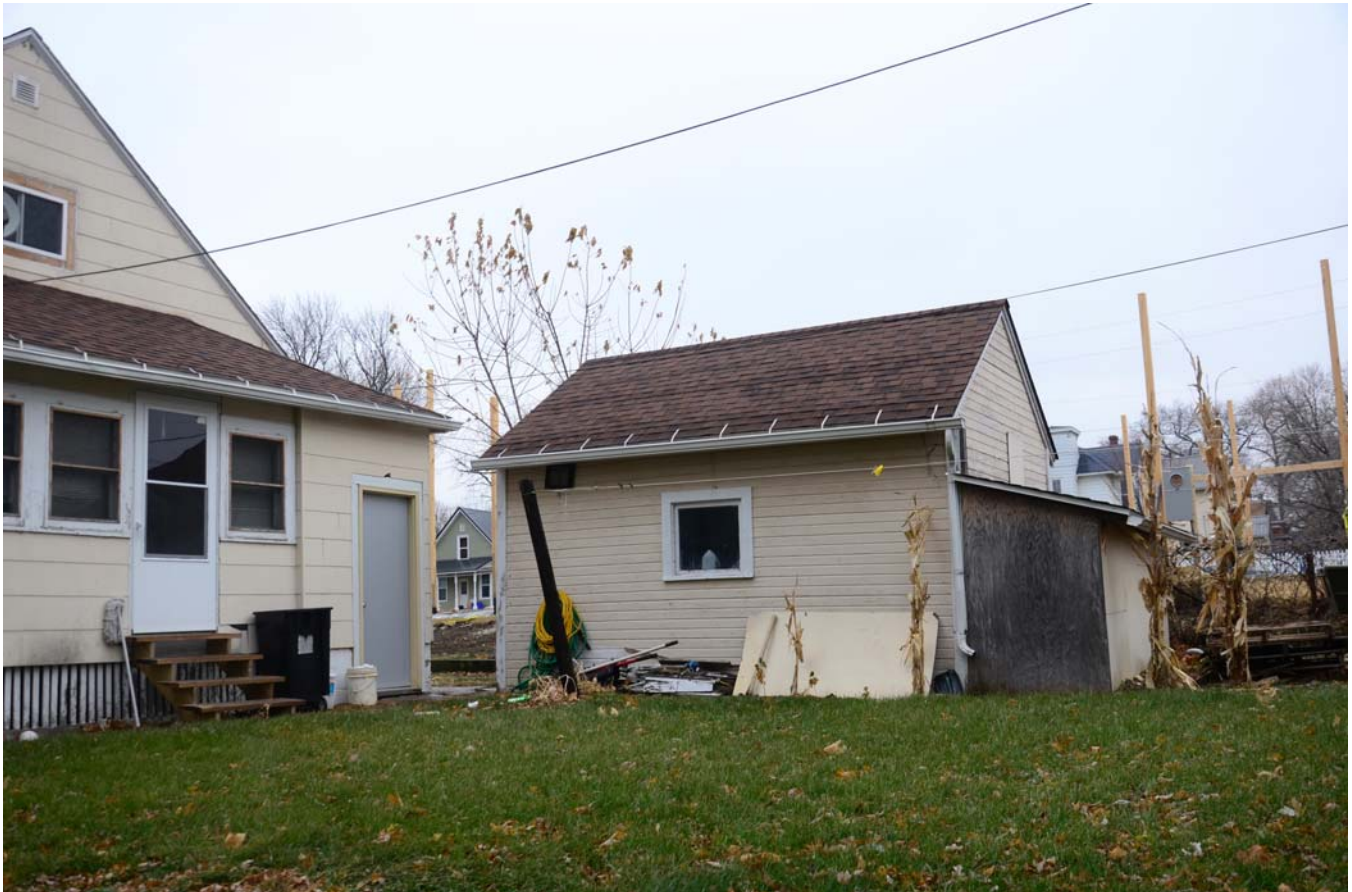
Photograph 92-00743-003 - Garage, looking northeast (December 2014)
