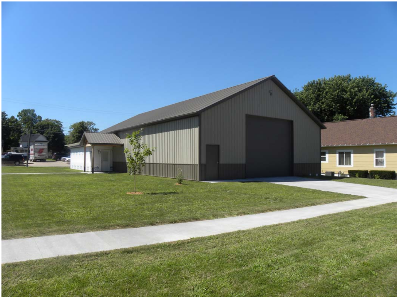
Photograph 92-00808-001 - Building, looking southwest (July 2015)
