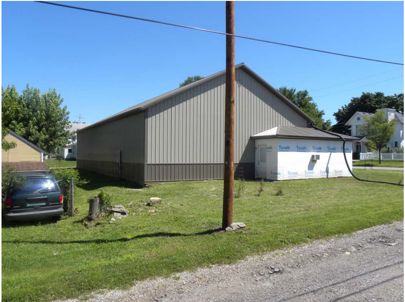
Photograph 92-00808-002 - Building, looking northeast (July 2015)
