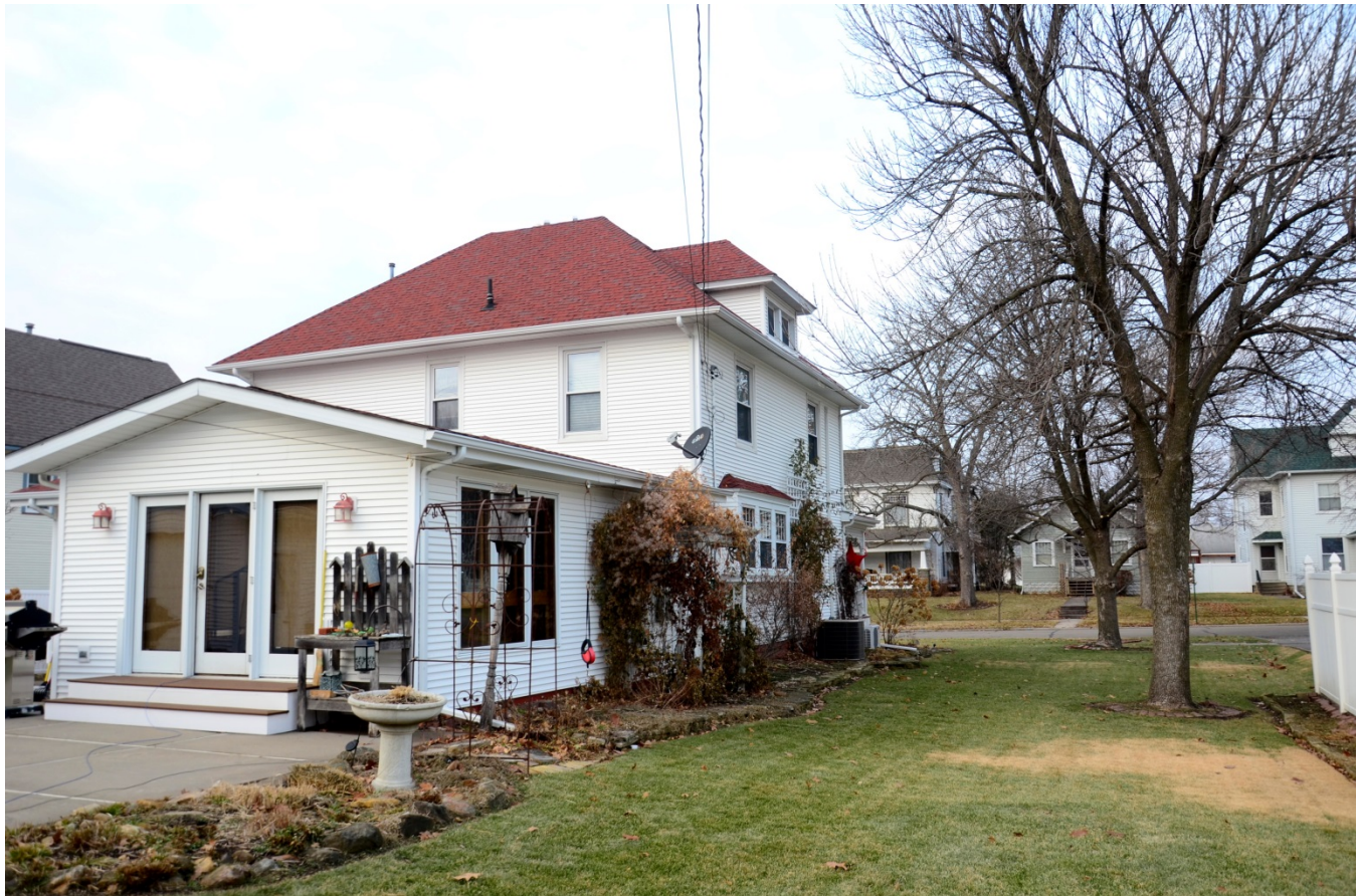
Photograph 92-00407-003 - House, looking northwest (December 2014)
