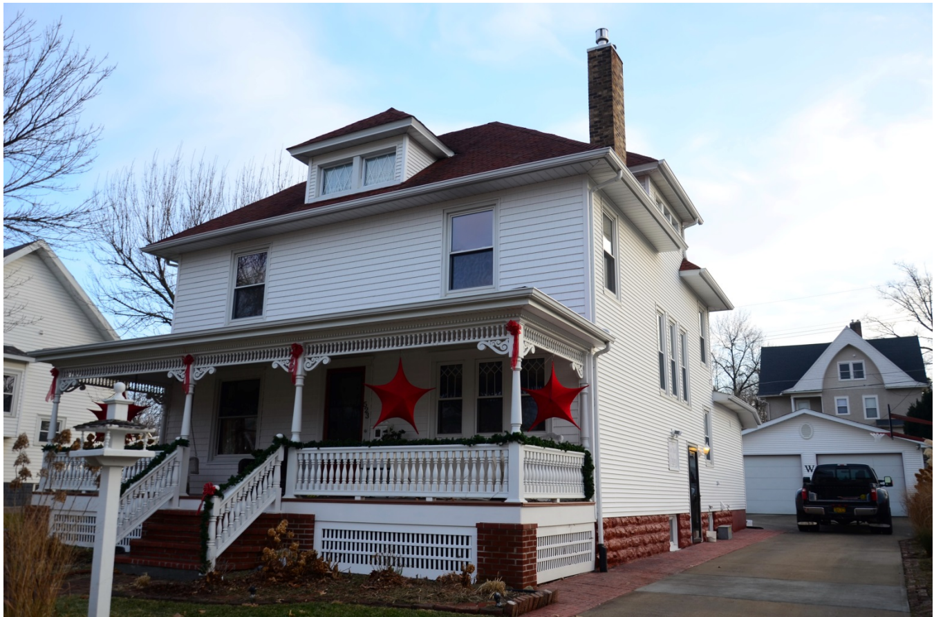
Photograph 92-00407-001 - House, looking southeast (December 2014)
