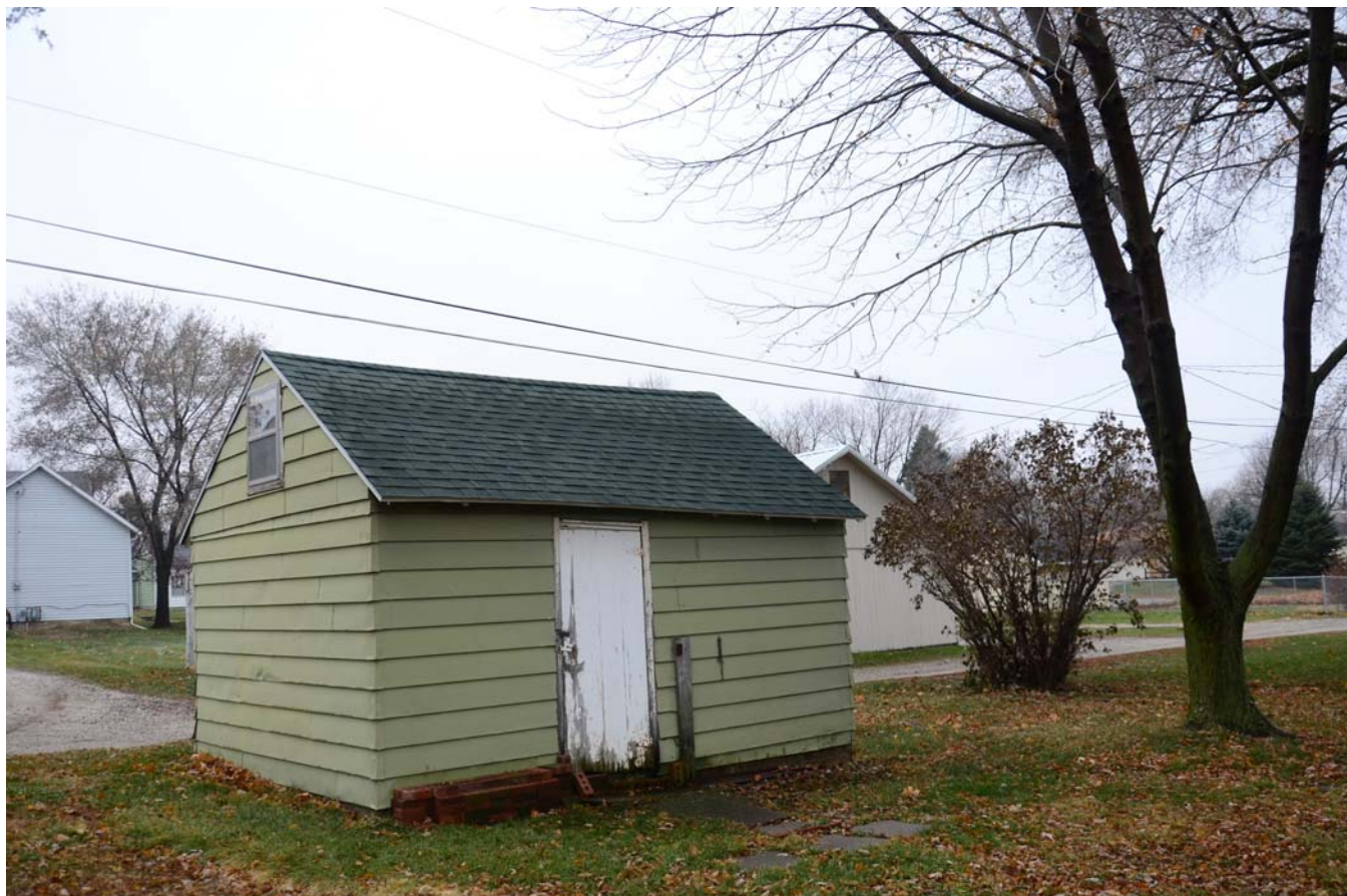
Photograph 92-00744-003 - Garage, looking southwest (December 2014)
