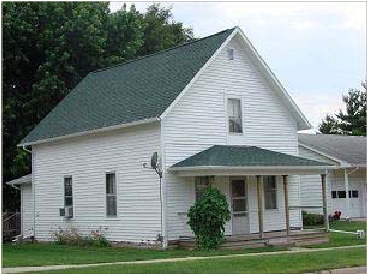
earlier photograph showing 2/2 wood windows
