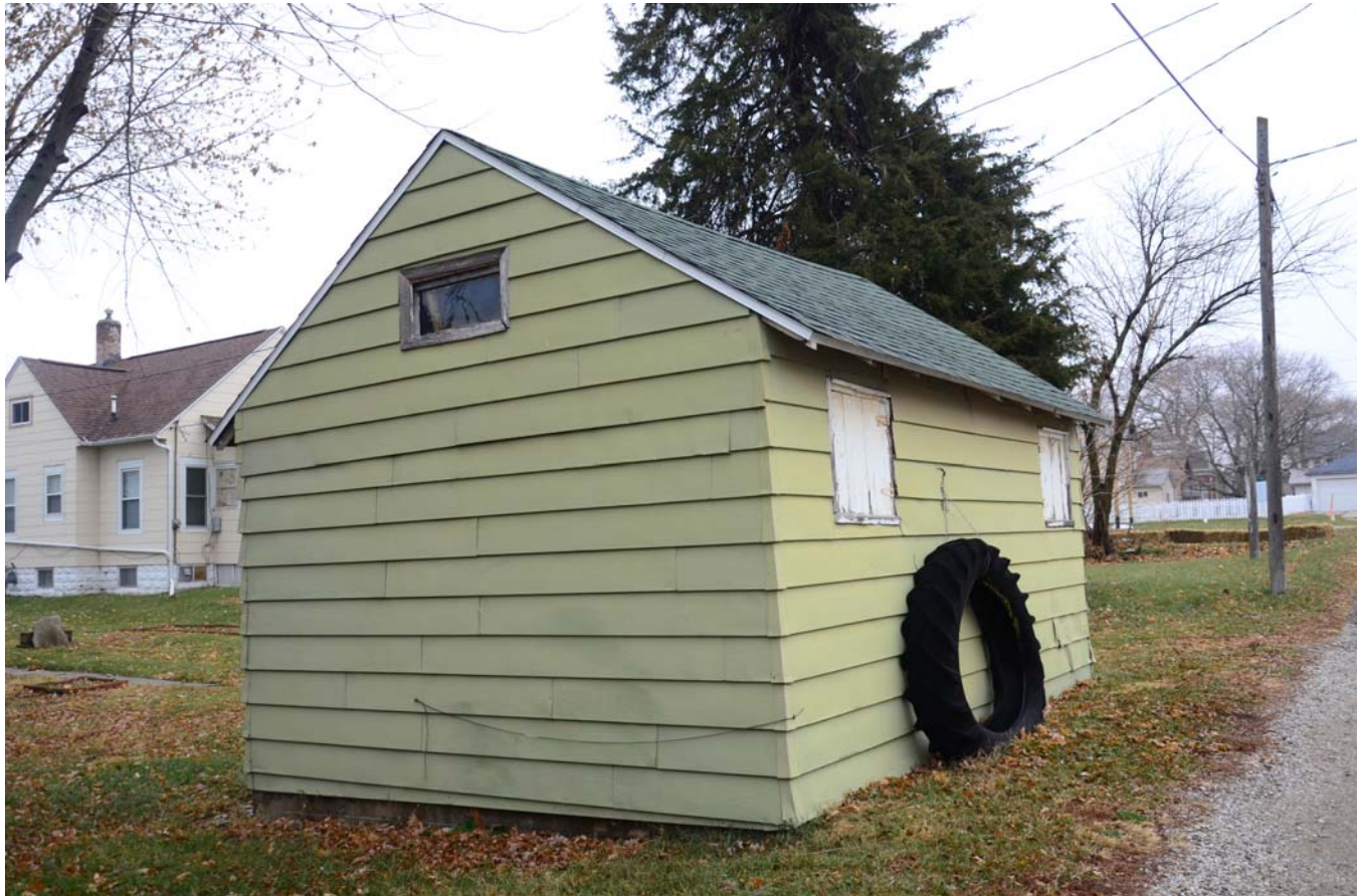
Photograph 92-00744-004 - Garage, looking northeast (December 2014)
