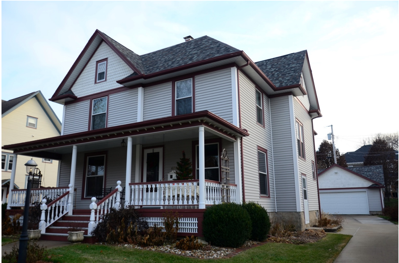
Photograph 92-00409-002 - House, looking southeast (December 2014)
