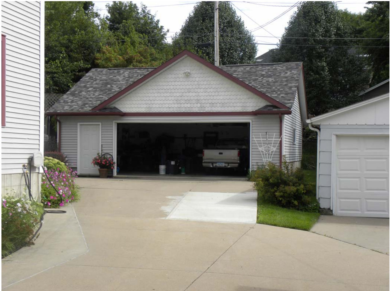
Photograph 92-00409-005 - Garage, looking south (July 2015)
