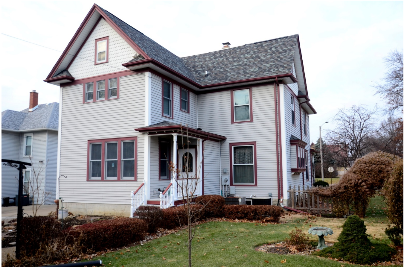
Photograph 92-00409-004 - House, looking northwest (December 2014)
