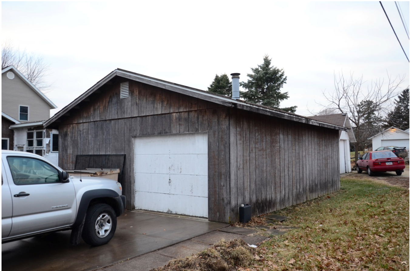
Photograph 92-00781-004 - Garage, looking southwest (December 2014)
