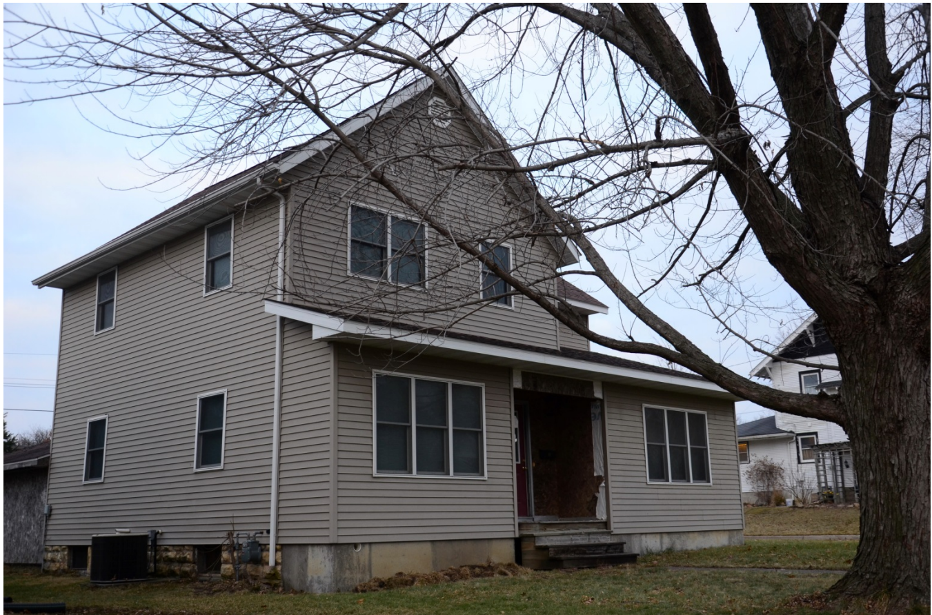
Photograph 92-00781-002 - House, looking northeast (December 2014)
