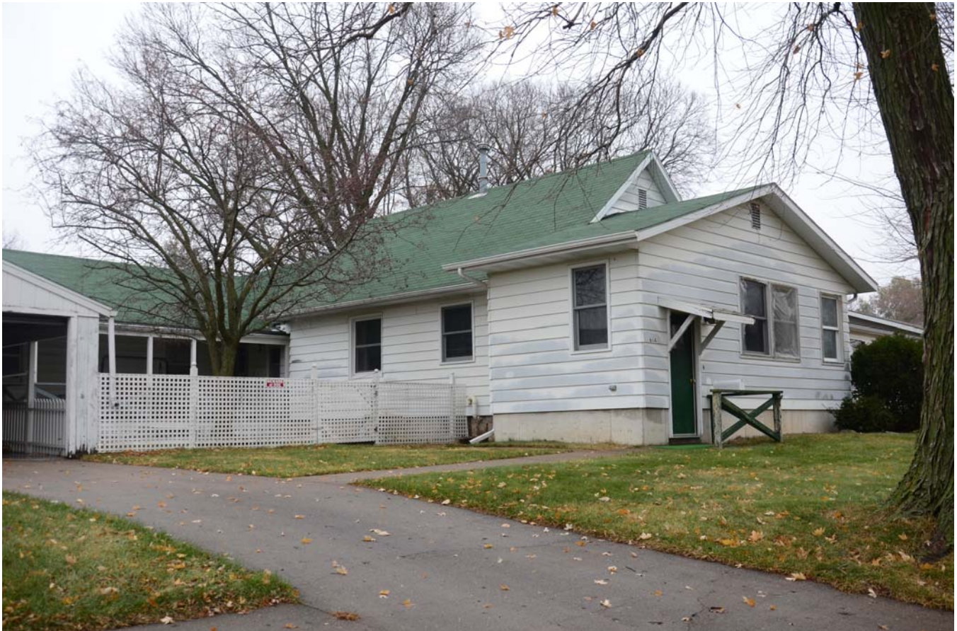
Photograph 92-00748-002 - House, looking northeast (December 2014)
