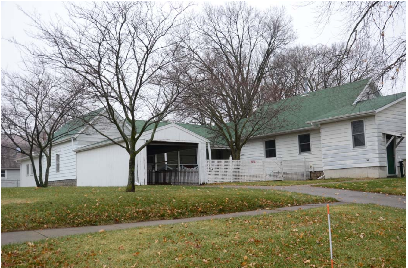
Photograph 92-00748-003 - House, looking northeast (December 2014)
