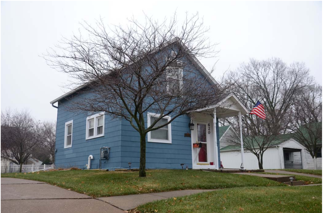
Photograph 92-00749-002 - House, looking northeast (December 2014)
